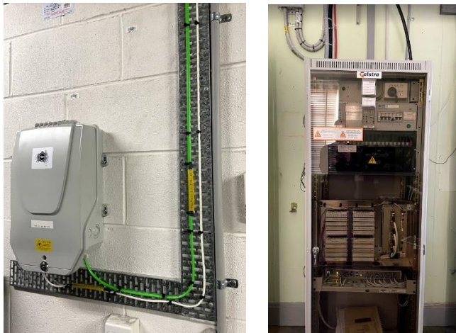
Figure 6 Telstra and NBN Co. Network Termination equipment
