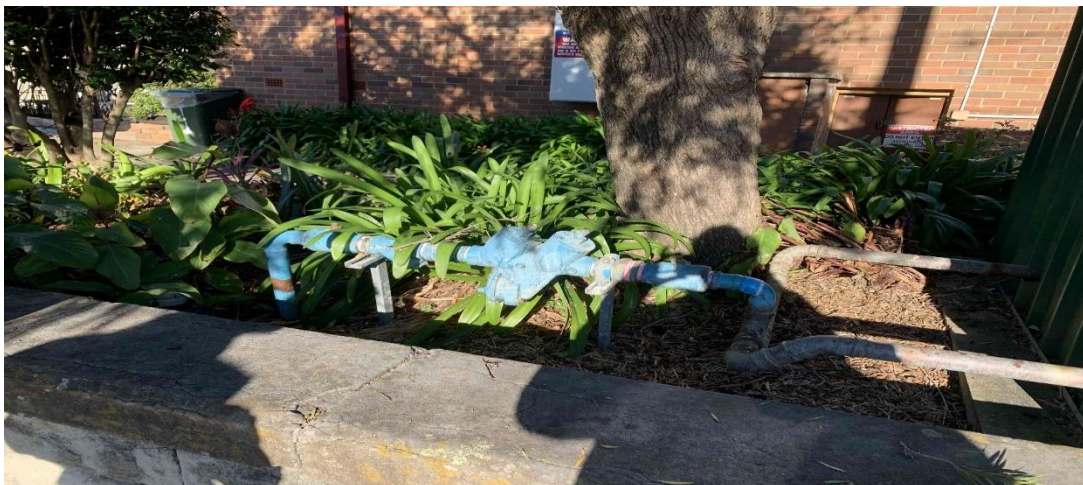
Photograph 5 – Secondary water meter located on Denistone Road, complete with backflow device
