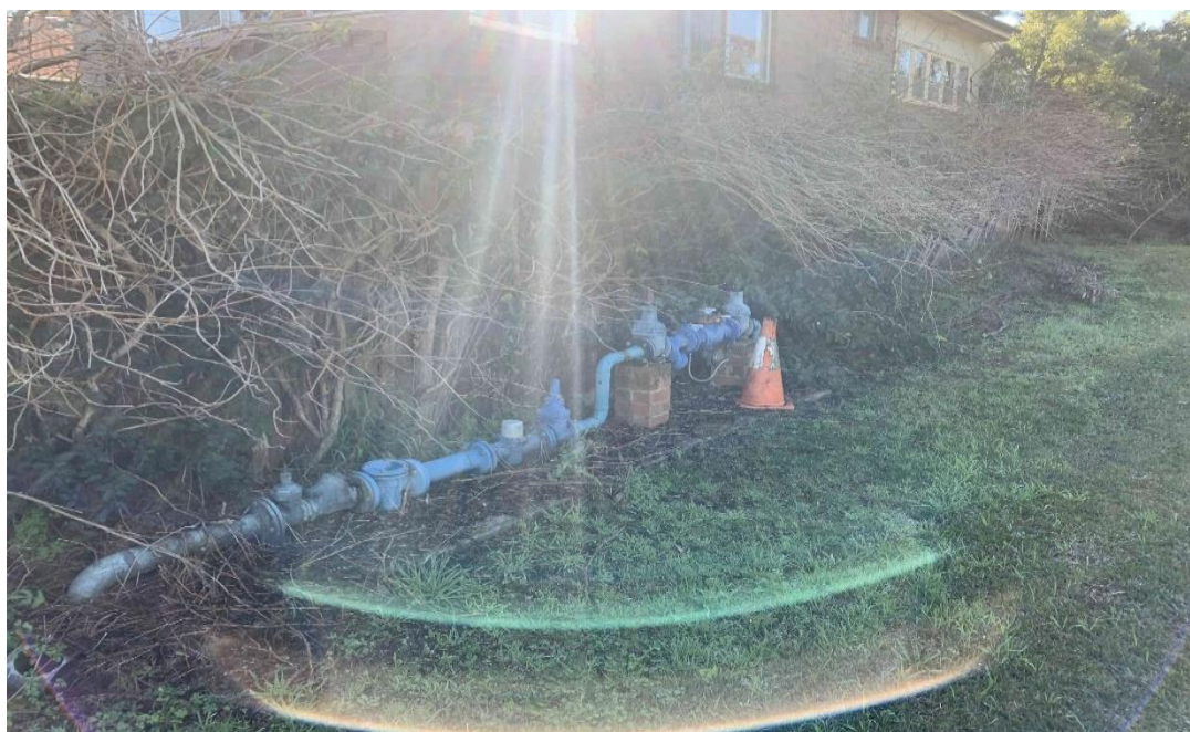
Photograph 1 - Potable water master meter located externally off Ryedale Rd – Serving the existing campus
