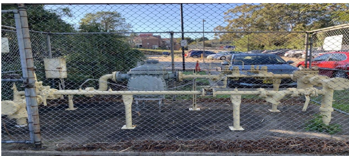
Photograph 6 – Existing site's master gas meter and regulator assembly
