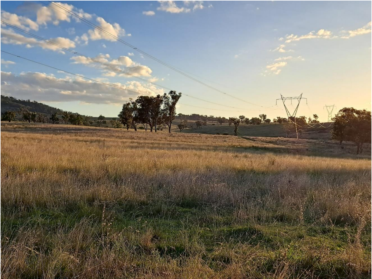
FIGURE 1-2 TRANSGRID'S EXISTING 330 KV ARMIDALE-TAMWORTH OVERHEAD TRANSMISSION LINE
