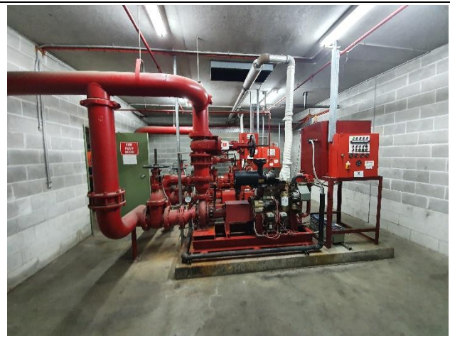
Photo 10: South east warehouse, pumphoom piping
