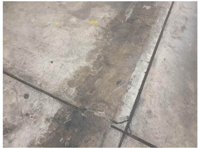
Photo 2: Internal, Main warehouse, slab expansion joint.
