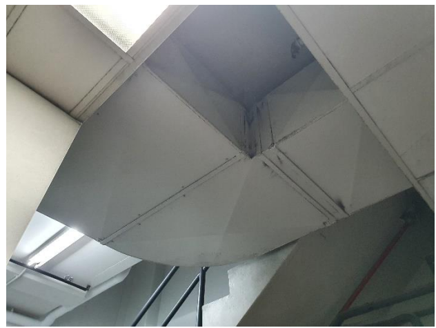
Photo 4: Main building, East office/store, ac ducting joints presumed positive for asbestos.
