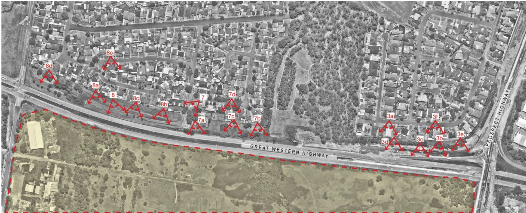
Figure 5b – Visual Receptor Locations (Residential area)
