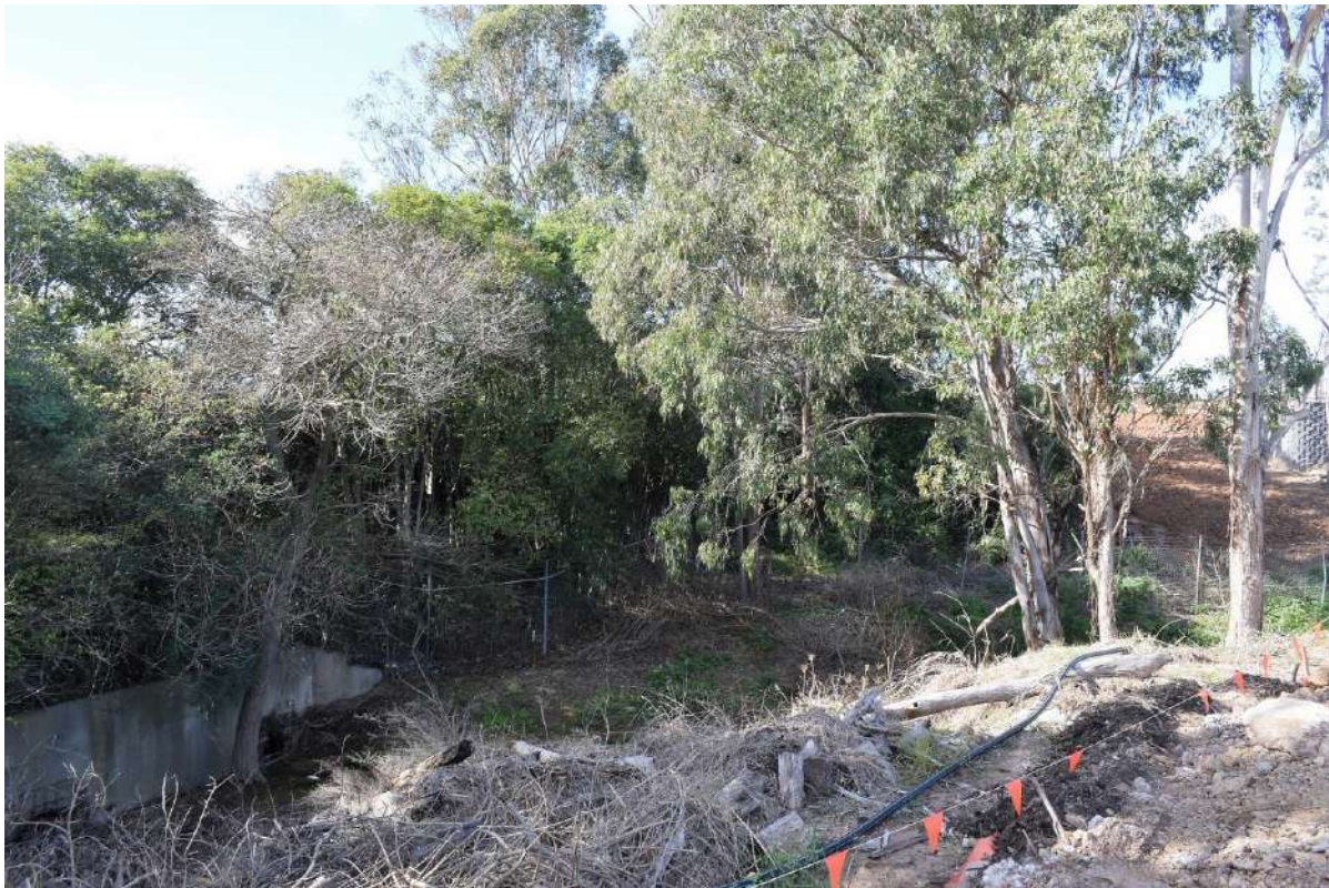
Conservation Area A: Looking NE, drainage swale with culvert on bottom left.
