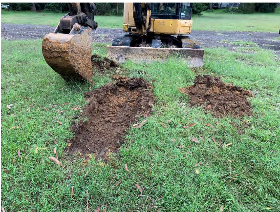
Photograph 18: TP28 advanced within a small fill platform adjacent to the asphalt area in the south of the Site.
