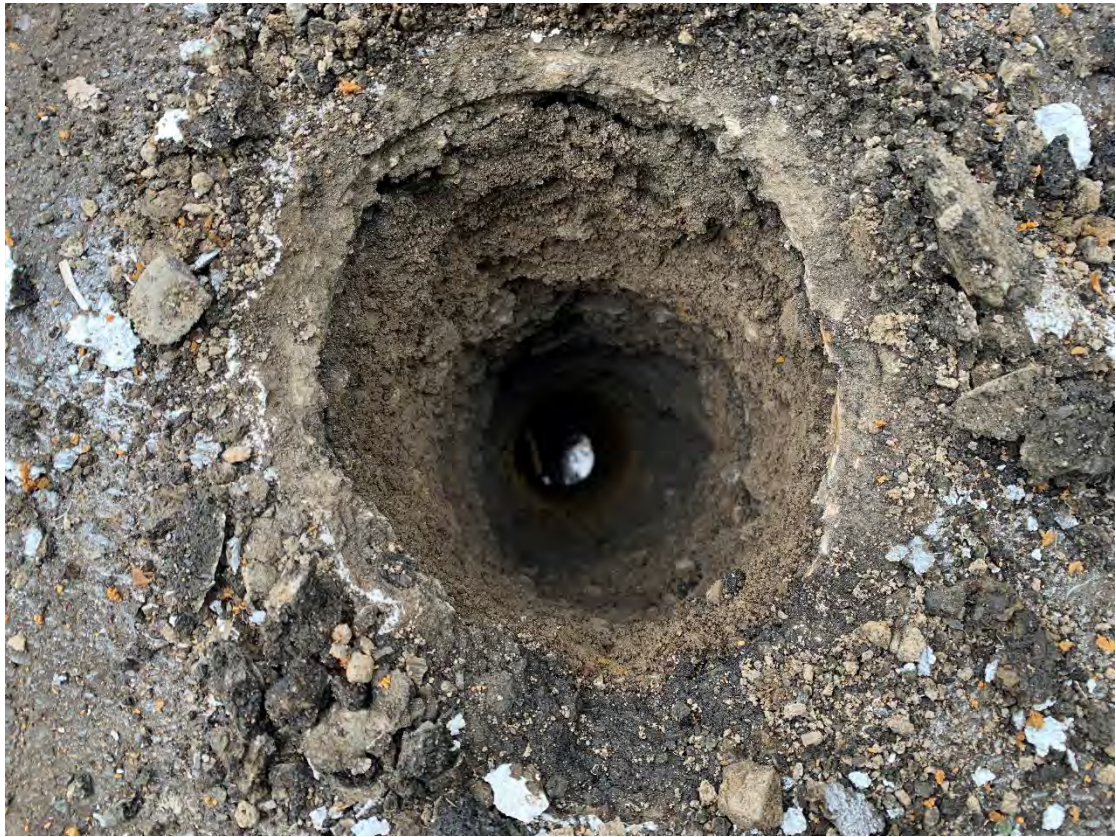
Photograph 3: Standing water observed in BH01S2
