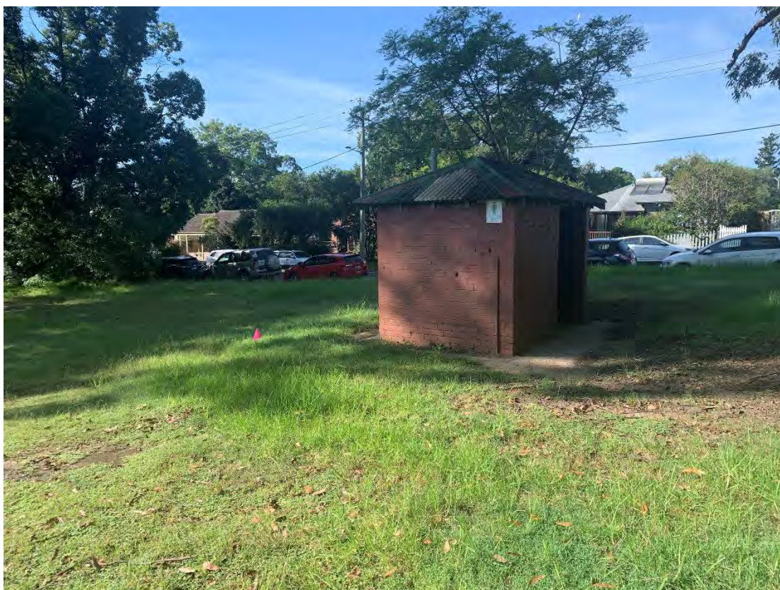
Photograph 7: Toilet building observed in the southern portion of the Site, note TP23 location indicated by the flag
