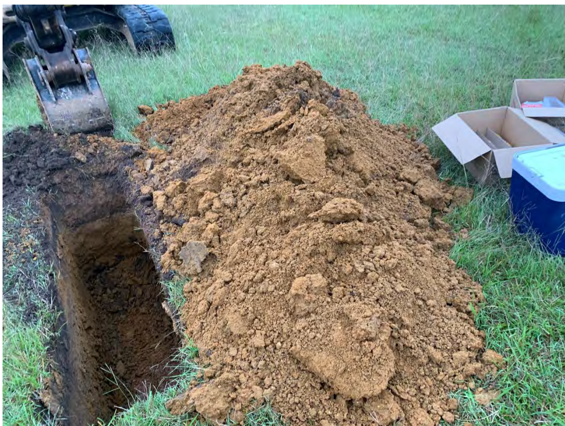
Photograph 17: TP24 spoil, note natural sandy clay strata.
