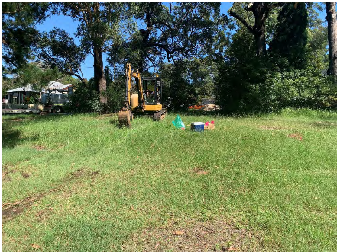
Photograph 10: 5t excavator used for test pitting, pictured in the proposed Shoalhaven Pre-school area. Note small fill platform.
