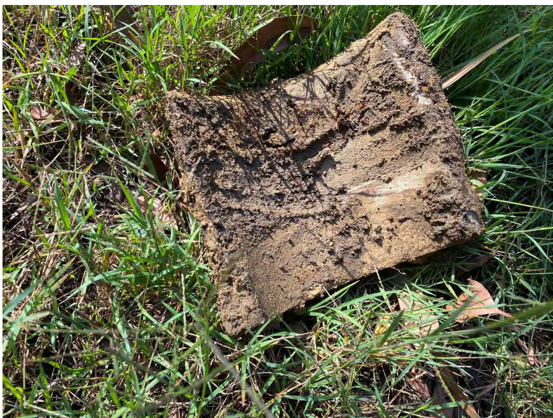
Photograph 14: Asbestos piping observed in TP20 spoil (TP20_0.4_PACM)
