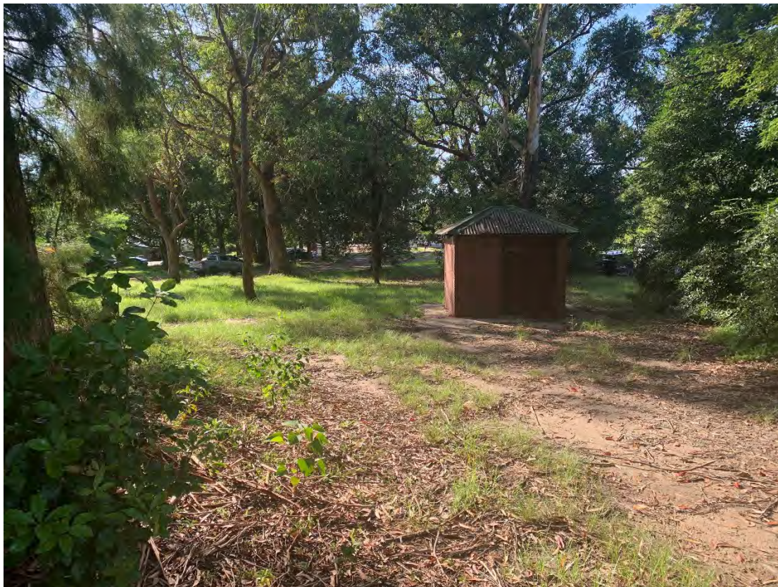
Photograph 8: Additional toilet building observed in the southern portion of the Site
