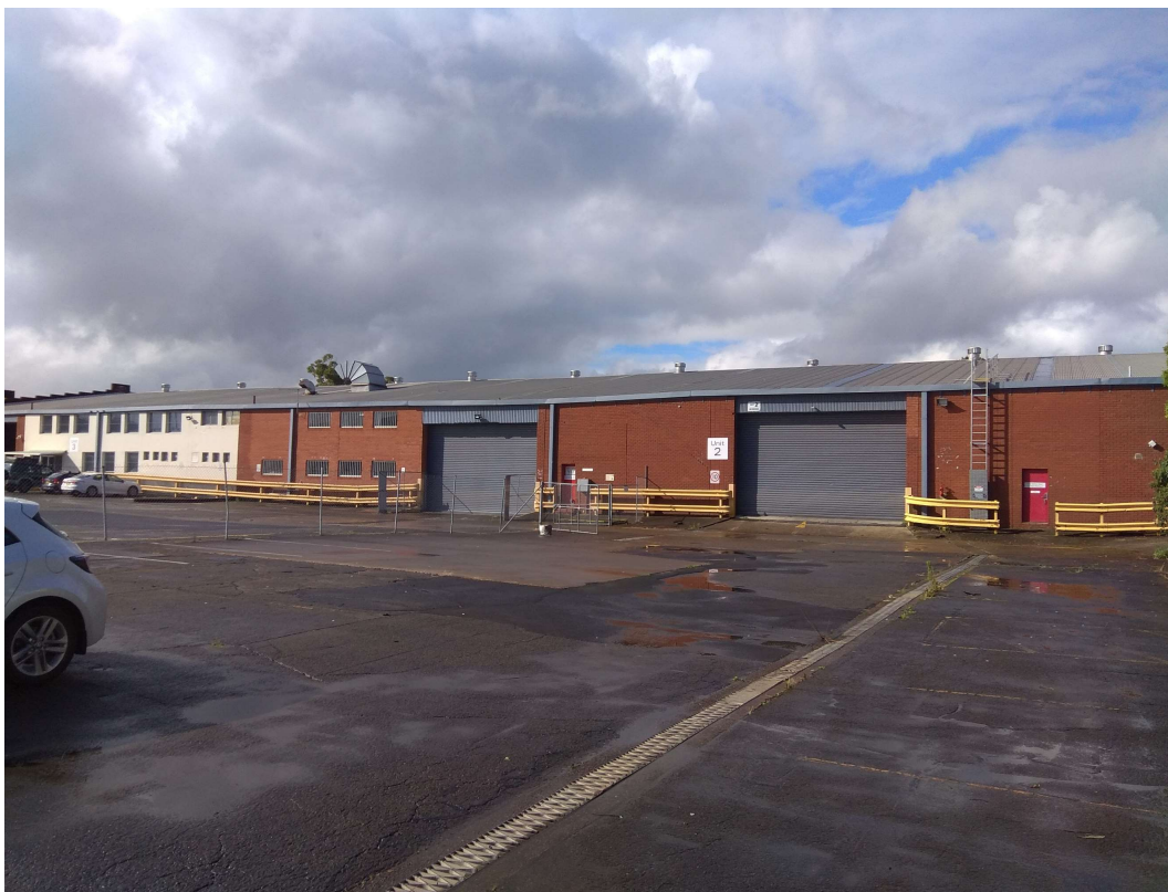
Photo 1: General site photo of the site near BH C looking towards the South East (11/07/2022)
