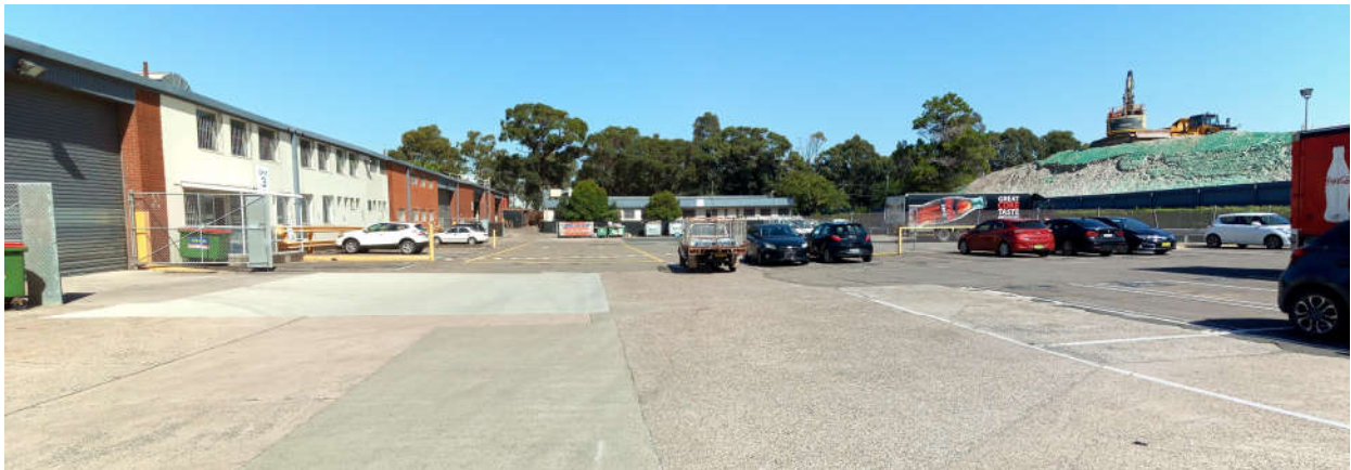
Photo 2 - General Site Conditions - View to the South from entrance
