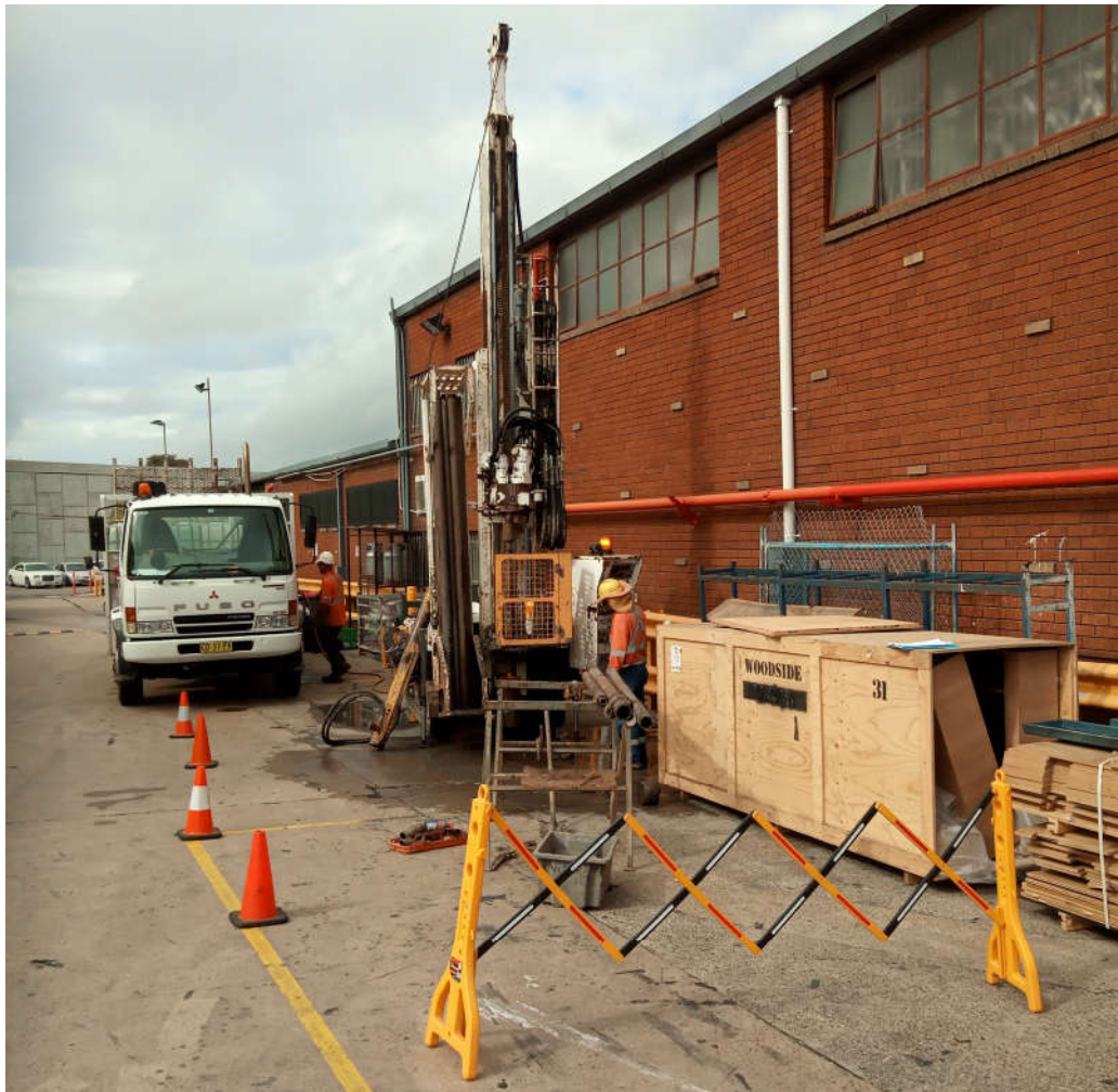
Photo 5 - Drilling rig and exclusion zone
