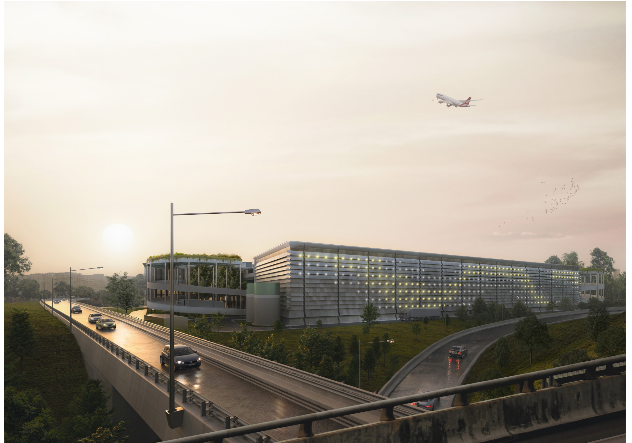
Artist impression - view from St Peters Interchange flyover to the north west
