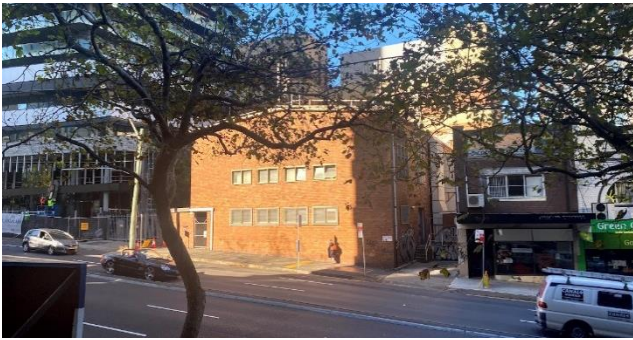
Figure 3 Existing Telstra Exchange Building from Pacific Highway to the north
