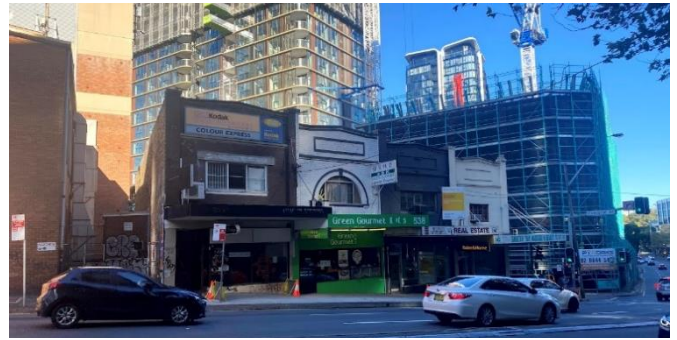
Figure 4 Existing retail/commercial buildings from Pacific Highway to the north
