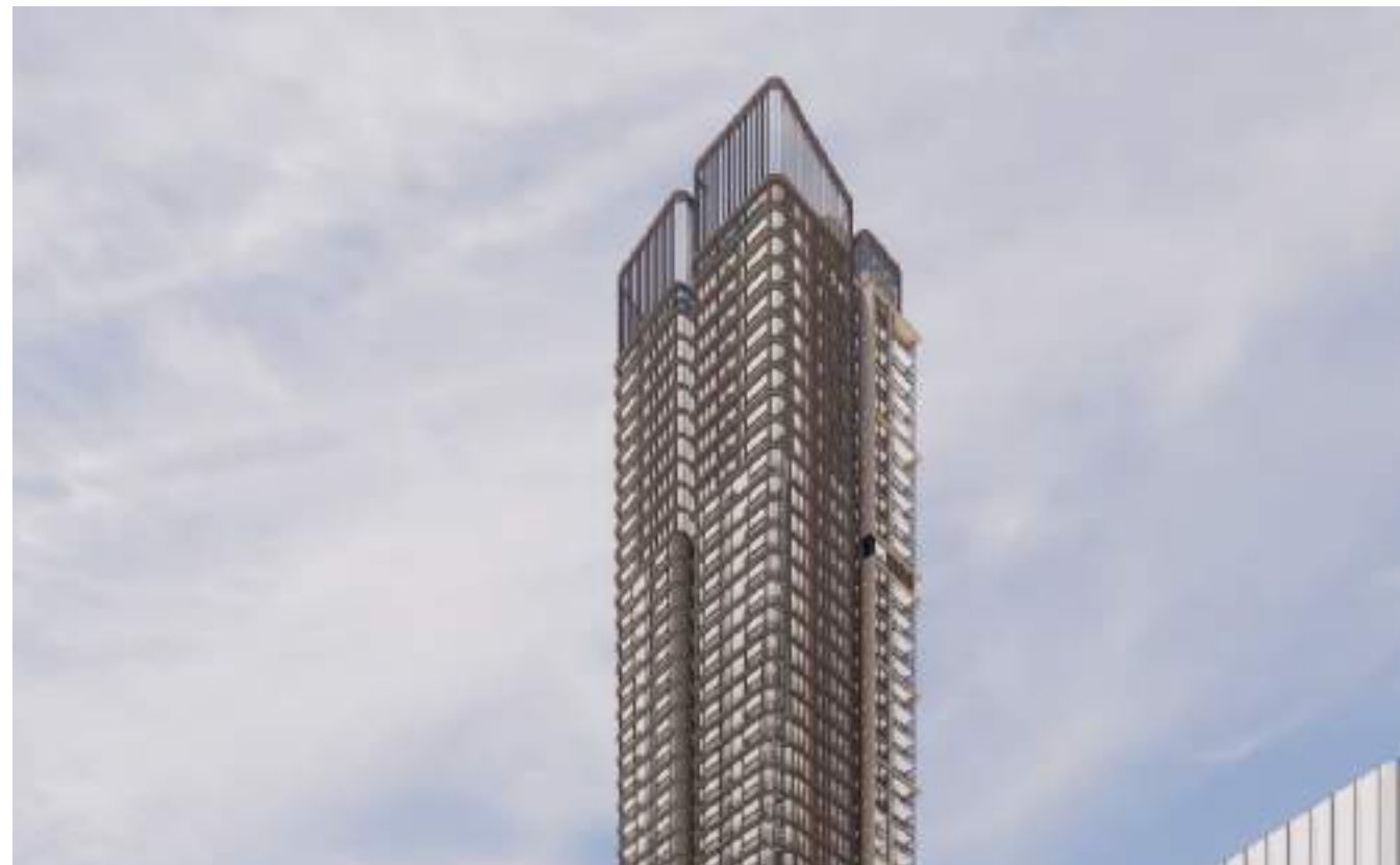
SSDA - NORTHERN VIEW OF ROOF ENCLOSURE
