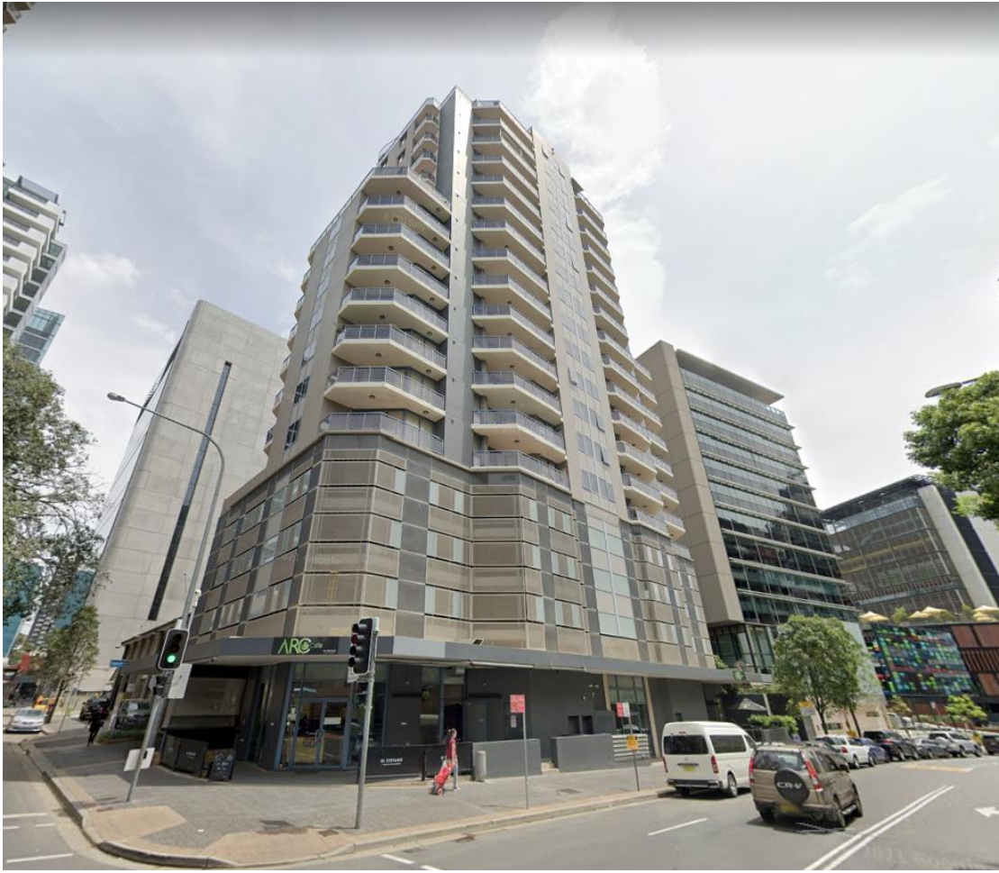
Photograph 4: Shows the adjoining building at 14 Hassall Street
