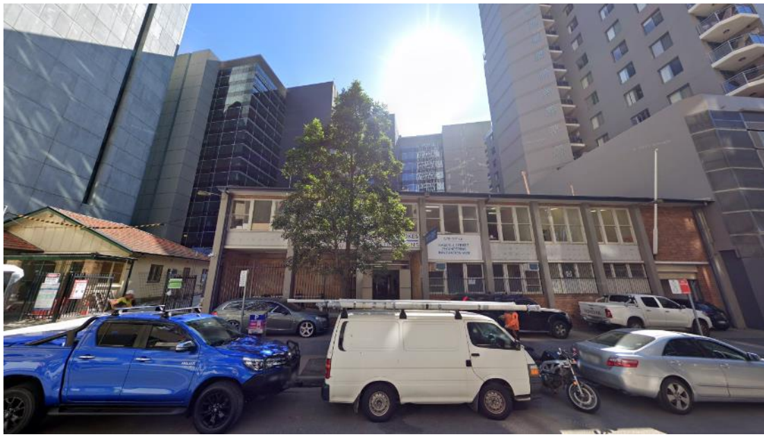
Photograph 1: Shows the site viewed from Hassall Street.
