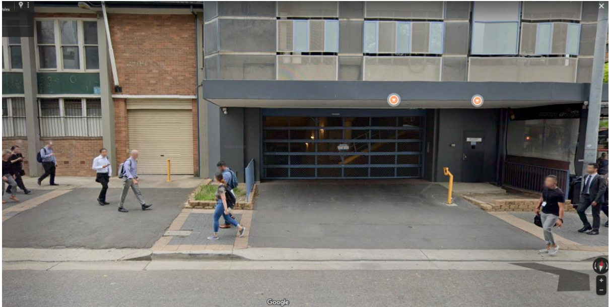
Figure 4 - 12 / 14 Hassall Street, Parramatta – Garden / Fencing Separator Island to Redirect Pedestrians for their safety
