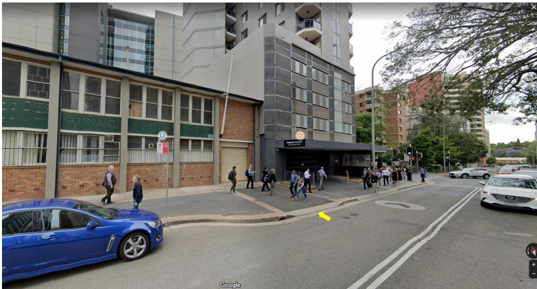
Figure 12 - 12 Hassall Street, Parramatta – Existing Eastern Boundary Single Lane Entry / Exit Access Driveway
