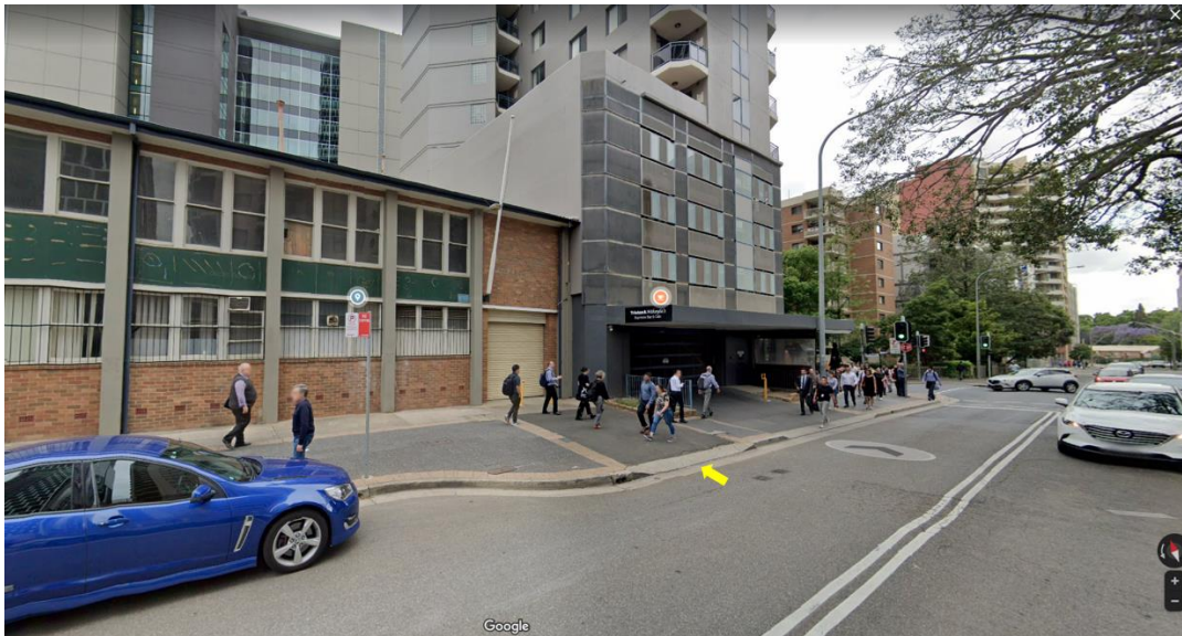
Figure 3 - 12 Hassall Street, Parramatta – Existing Eastern Boundary Single Lane Entry / Exit Access Driveway
