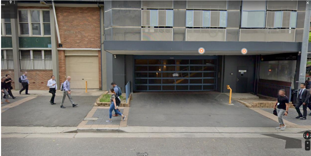
Figure 13 - 12 / 14 Hassall Street, Parramatta – Garden / Fencing Separator Island to Redirect Pedestrians for their safety
