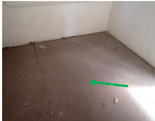
Photo 5: Residence – non-asbestos containing red vinyl flooring to the northwest room
