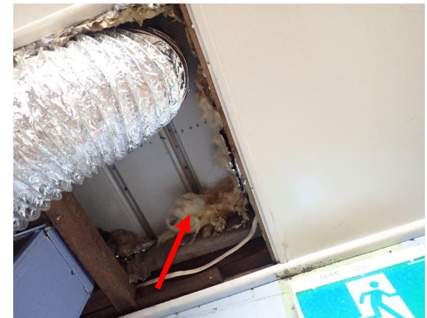
Photo 24: PCYC – assumed SMF insulation within the north ceiling cavity of the garage
