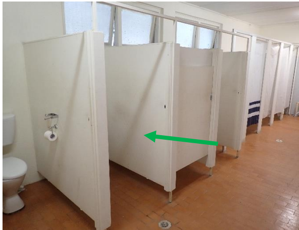
Photo 19: PCYC – non-asbestos containing compressed fibre cement cubicle partitions to the northeast male toilets
