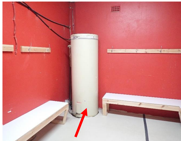
Photo 23: PCYC – assumed internal SMF insulation to the hot water system in the male change room
