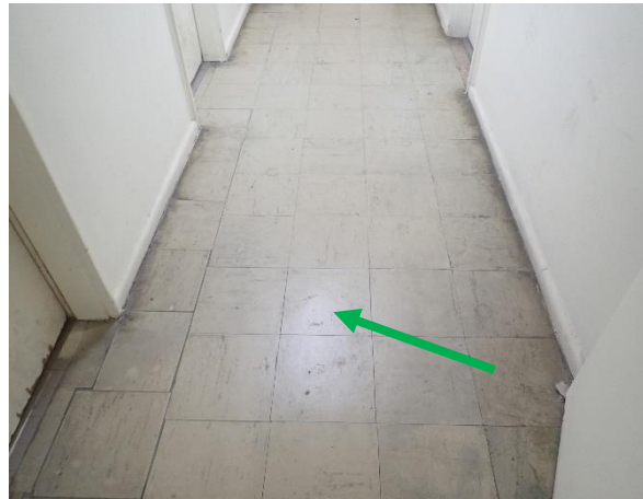
Photo 20: PCYC – non-asbestos containing white vinyl floor tiles to the amenities corridor in the south portion
