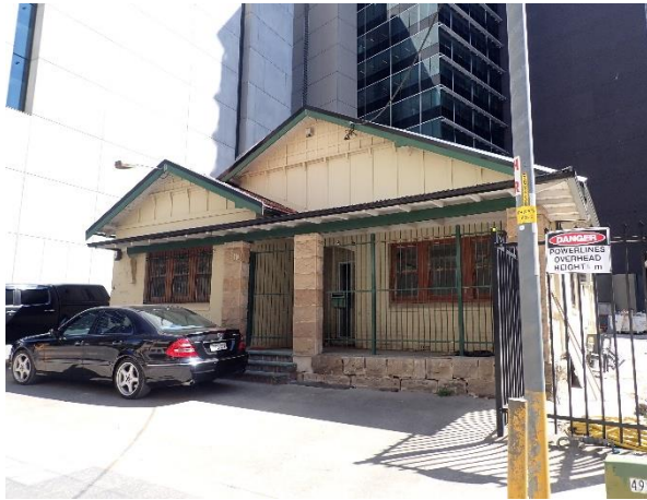
Photo 1: Overview of the Residence
