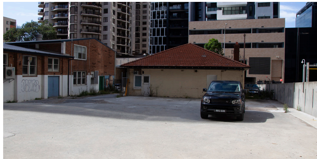
View south to Hassall Street
