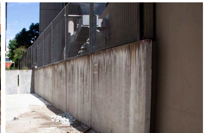
Existing northern boundary fence
