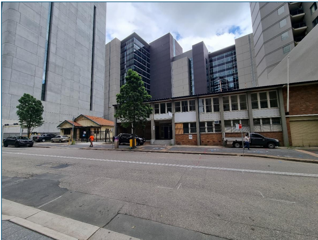
Photograph 2: Showing the former Police Youth Club building and cottage
