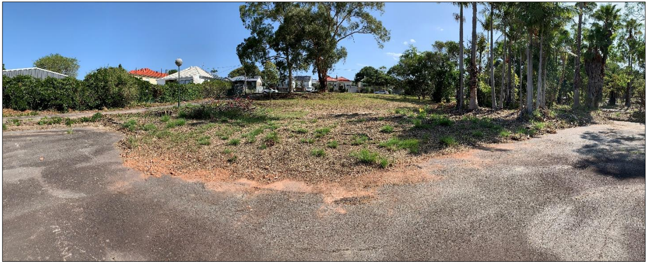
Photo 31: Former administration building located adjacent to eastern entrance, comprising concrete slabs, brick footings and terraced garden beds, looking south.
