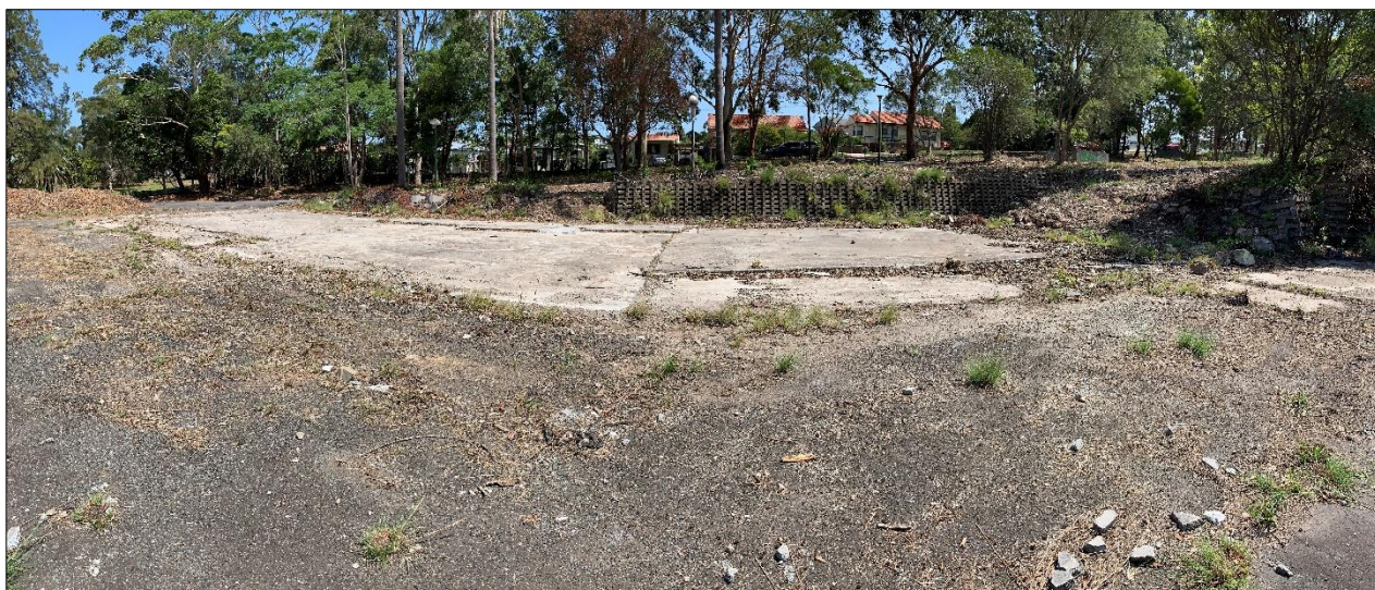
Photo 15: Central portion of site comprising a concrete and asphalt sealed hardstand area associated with the former chemical shed, potting shed and machinery shed, looking south. Note: Crib-lock wall in the background
