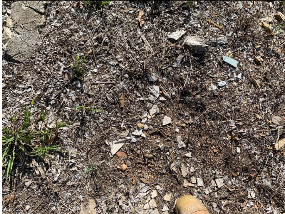
Photo 39: Demolition waste at the surface of former classrooms footprint including concrete, bricks, sandstone, pavers, PVC, agricultural pipe, PVC, metal and areas with multiple fibro fragments.
