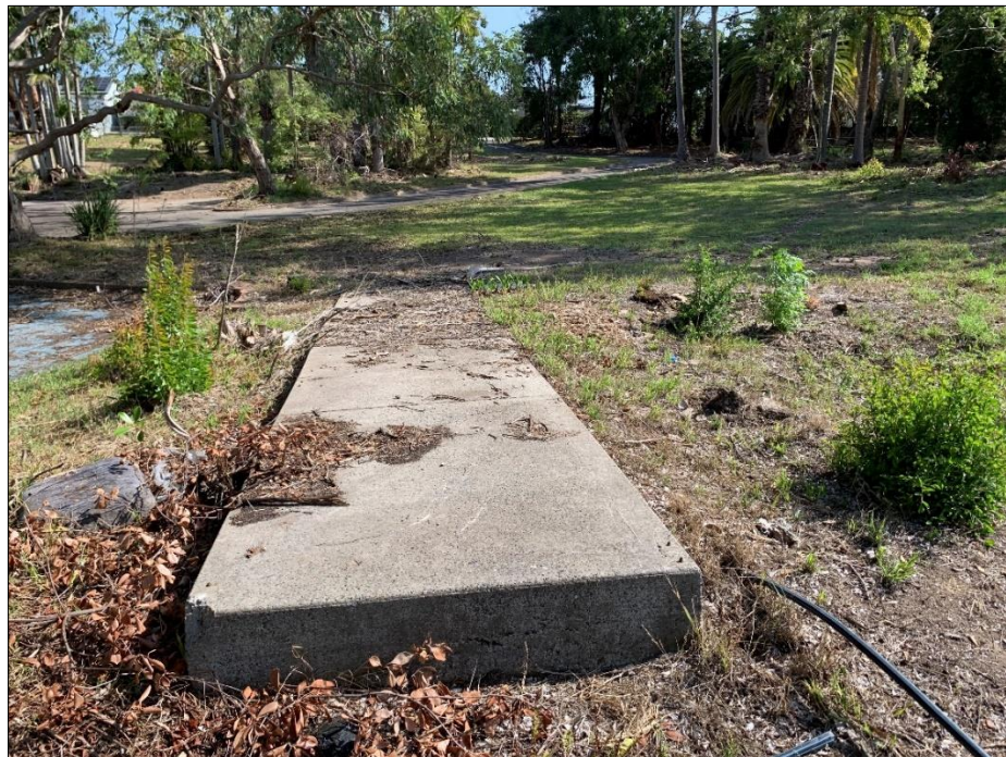
Photo 38: Area north of the driveway (former classrooms) comprising a grassed area with remnants of former building slabs and footings.
