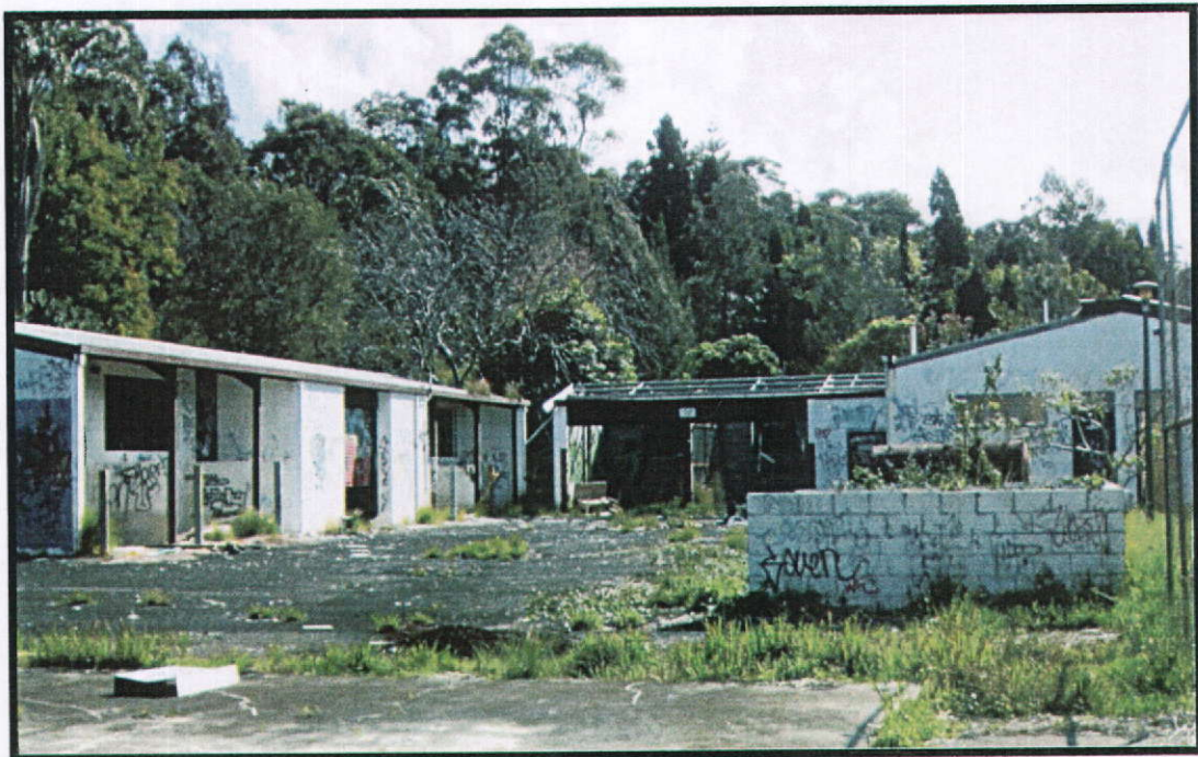
Photo 3: Eastern elevation of Buildings 1, 2 and 3 as identified on the Plan of Demolition.
