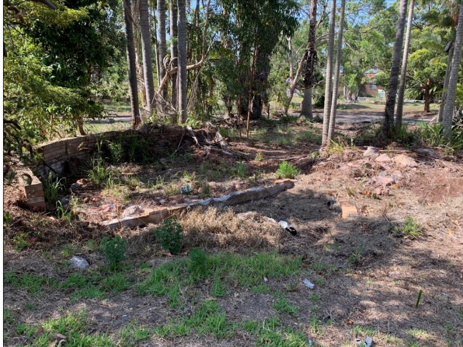
Photo 29: Partially demolished pool and water feature, adjacent to the central driveway entrance, looking north east.
