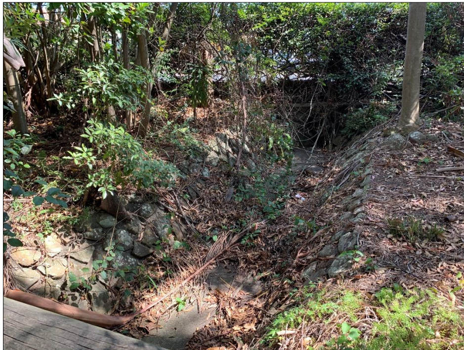
Photo 28: Open stormwater drain, constructed with battered natural rock/cement walls and a concrete base located at the eastern end of the garden area, looking south.
