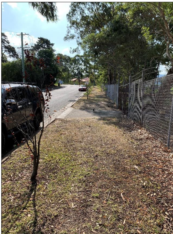
Photo 45: Fibro fragments observed on surface of road shoulder along Tiral Street, looking west.
