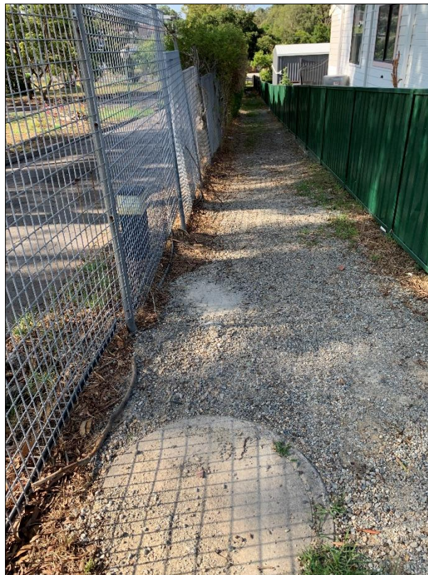
Photo 42: Easement to the east of the site comprises a gravel filled surface with the occasional manhole, looking north.
