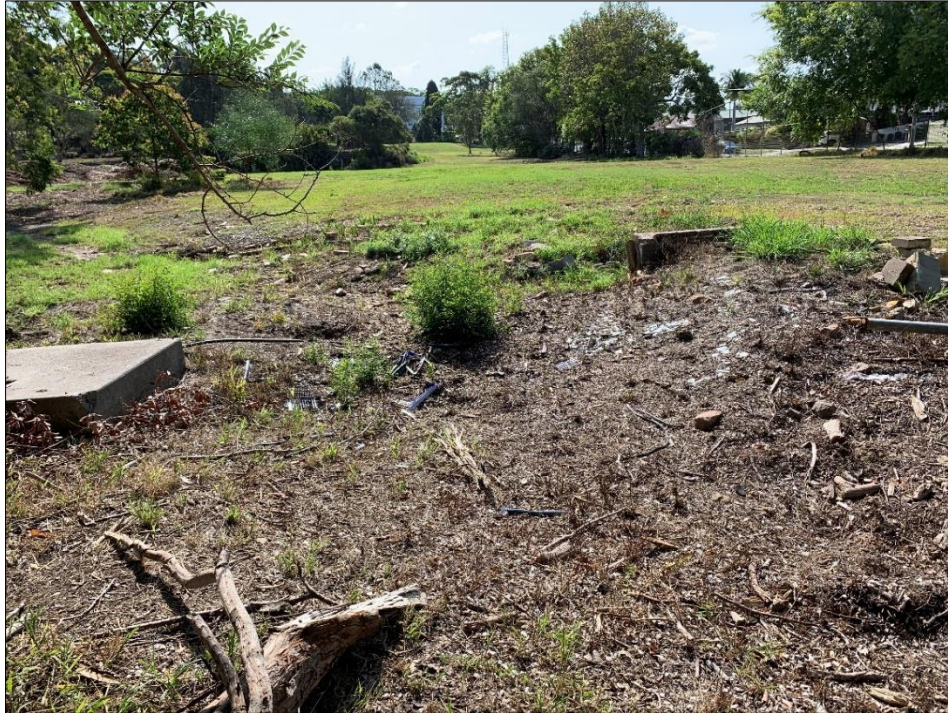
Photo 37: Area north of the driveway (former classrooms) comprising a grassed area with remnants of former building slabs and footings.
