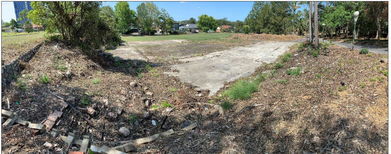
Photo 23: Partially demolished rock retaining wall located in the south western corner of the hardstand area, looking north east.
