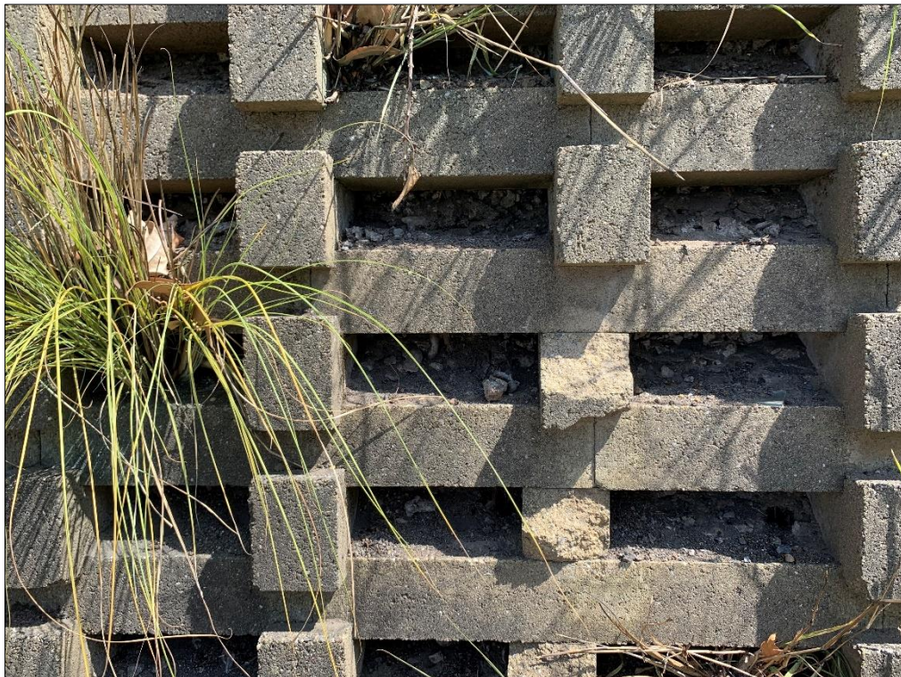
Photo 2: Southern crib-lock retaining wall comprising soil and ash, looking south.
