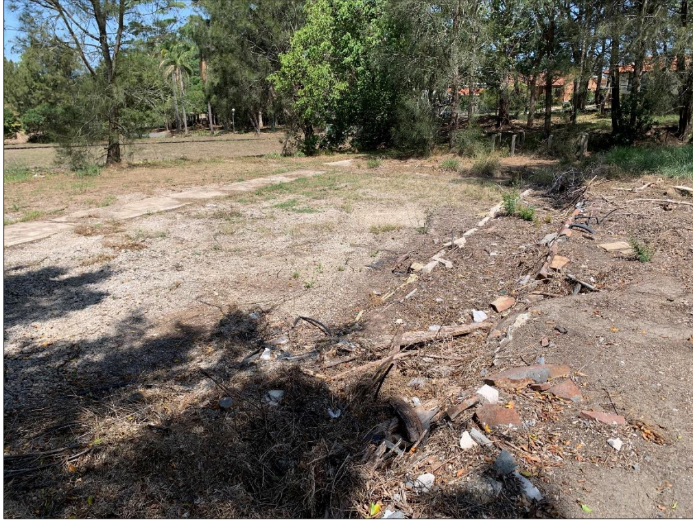
Photo 13: Former greenhouse area comprising blast furnace slag and gravel, looking east.
