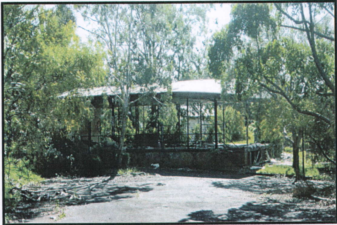
Photo 2: Eastern elevation of Building 7 as identified on Plan of Demolition.
