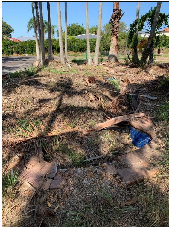
Photo 30: Backfilled inground pool, adjacent to the central driveway entrance. Note: Fibro sheeting fragments at surface
