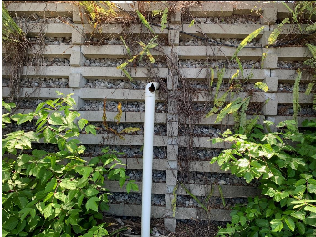
Photo 1: Western crib-lock retaining wall comprising blast furnace slag, looking west.
