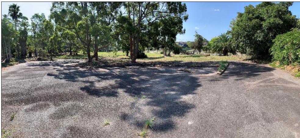
Photo 34: Asphalt sealed driveway and carparking area situated to the north of the former Administration building, looking north.
