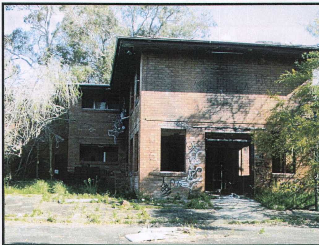
Photo 1: Northern Elevation of Building 8 as identified on Plan of Demolition.
