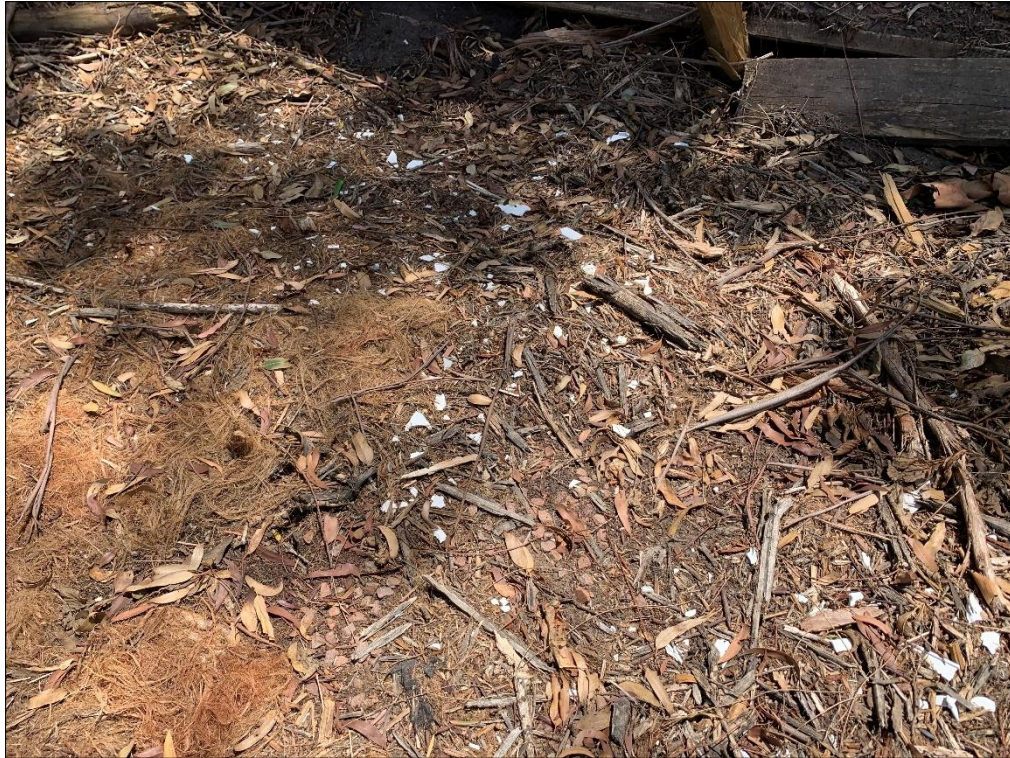
Photo 5: Fibro fragments at the base of the retaining wall adjacent to the former bowling green.
