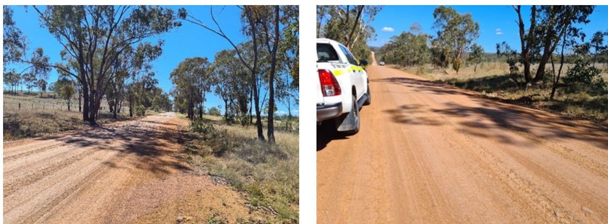
Figure 2-6: Wollara Road looking north (left) and south (right)
