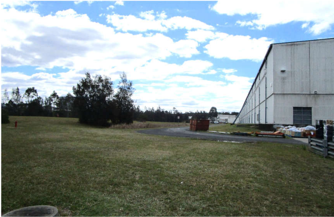
PHOTOGRAPH 1 – WESTERN WAREHOUSE ADDITION LOCATION
