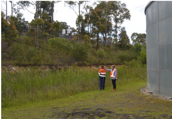
Figure 15. View of cut into slope, rear of fire tanks, northern boundary.
