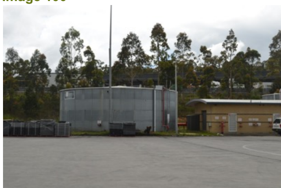
Figure 19. Fire tanks at north end of site. Image 100
