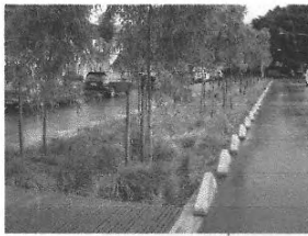
Car Park Centre Median Bioretention as landscape features to collect runoff and percolates through prescribed soil filtration media that is densely vegetated. Research by CRC indicates best practise treatment of runoff using bioretention results in 25-30% reduction in flow volume for all events under Q3mth (through wetting and evapotranspiration)
