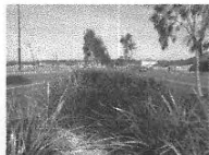
Heavily Vegetated Swale – Linear Wetland Systems to convey flow in lieu of pipes and provide treatment prior to discharge or entering storage.
