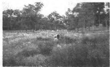
Heavily Vegetated Swale – Linear Wetland Systems to convey flow in lieu of pipes and provide treatment prior to discharge or entering storage.
