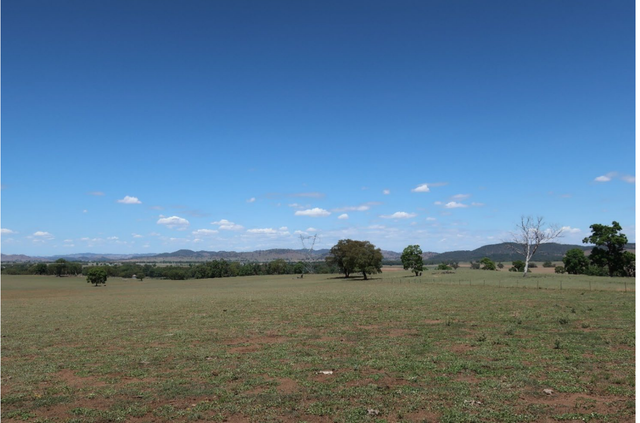
Photograph 2.6 – View of existing 330kV transmission line within project area looking south.
