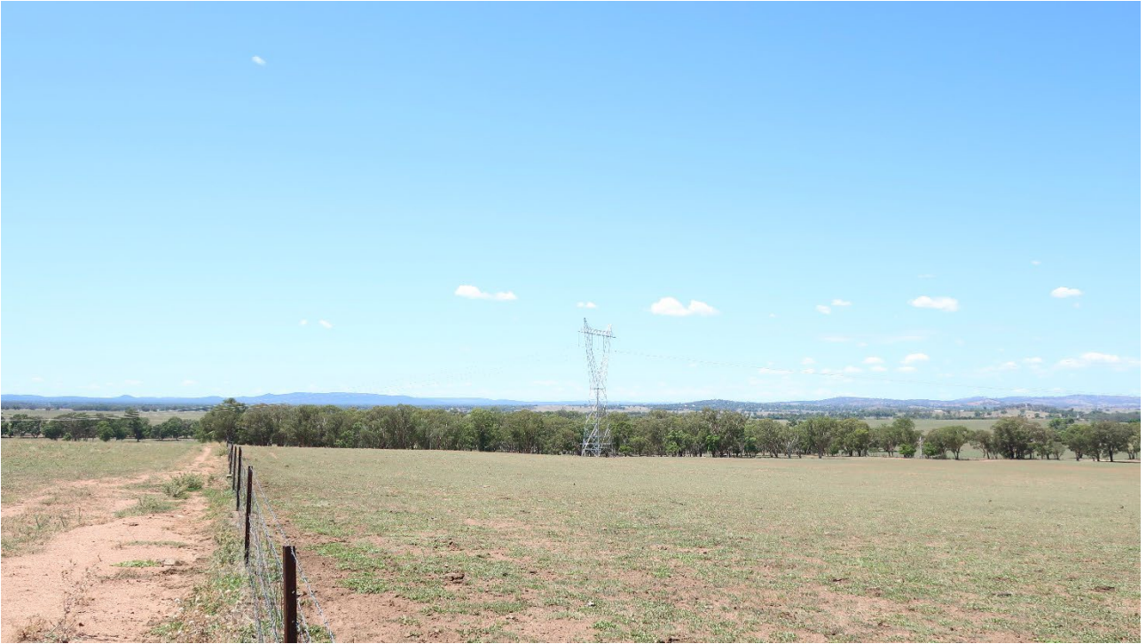
Photograph 2.5 – Views of existing 330 kV transmission line within project area looking east.
