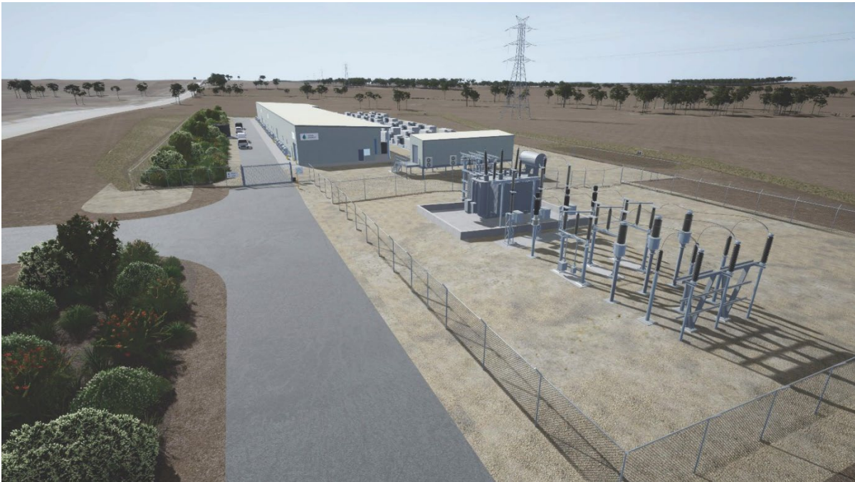
Figure 3.3 – Example view of VEA’s Wandoan South BESS site
