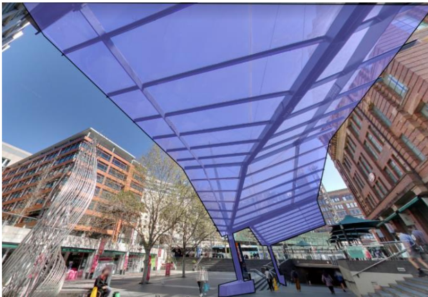
Figure 4.2.2b – Elevation view of awning and south retail demolition works shown in purple.
