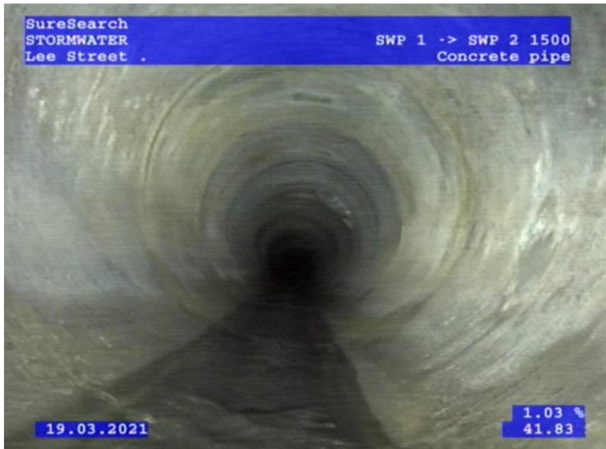
Figure 7 – Existing 1500mm Stormwater Culvert CCTV (SureSearch, 2021)
