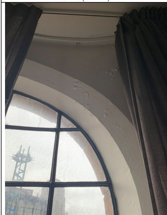
Figure 5 – Detail view to minor paint bubbling to window interior within Unit 38 (Level 3).
