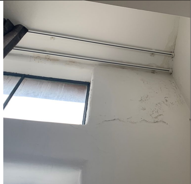
Figure 8 – Detail view to minor water damage and mould within Unit 73 (Level 5).
