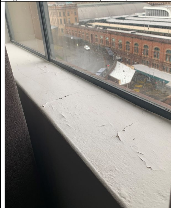
Figure 9 – Detail view to minor paint flaking to window interior within Unit 77 (Level 5).
