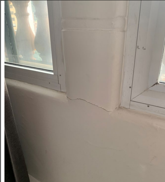
Figure 7 – Detail view to minor paint cracking to original fabric wall in Unit 62 (Level 4).
