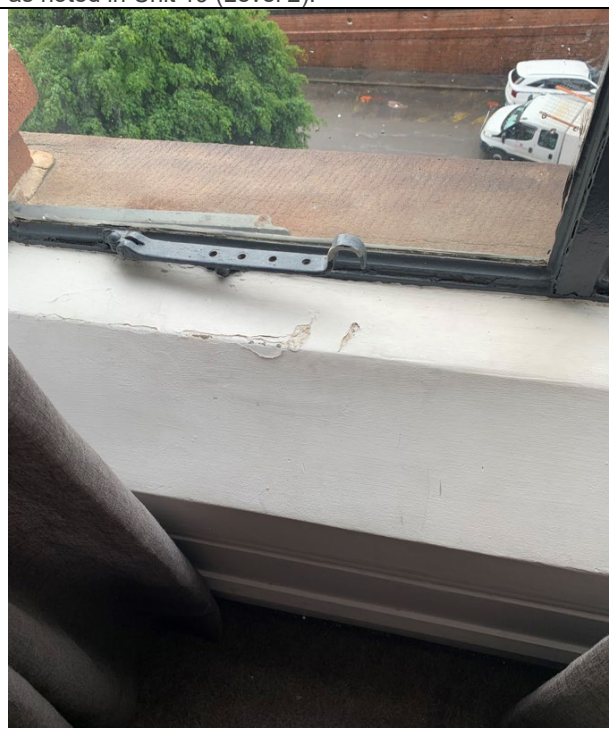
Figure 6 – Detail view to minor paint flaking and peeling to window interior within Unit 42 (Level 3).
