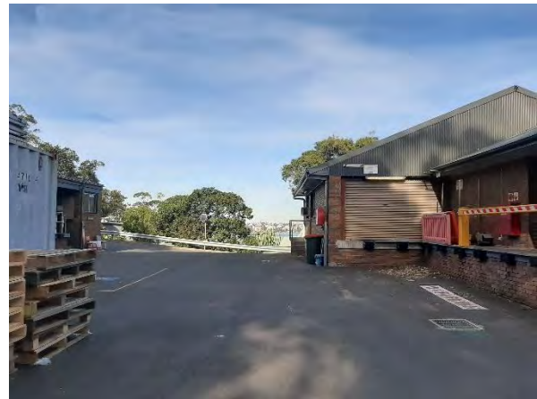
Figure 29 – Back of house facility. aspect: south.
