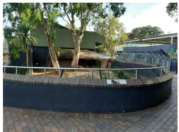
Figure 8 – Existing reptile house with excavated enclosure. Aspect: west.
