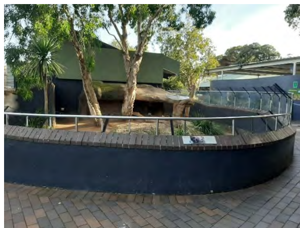
Figure 31 – Existing reptile house with excavated enclosure. Aspect: west.
