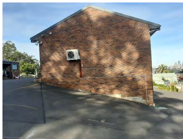
Figure 4 – Building cut into modified landscape. Aspect: south.
