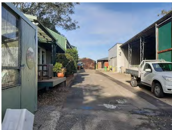
Figure 3 –General view, back of house area, with services evident. Aspect: north.
