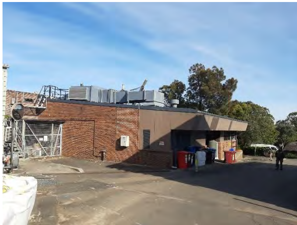
Figure 5 – Back of house facility. Aspect: south west.
