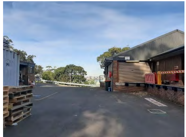
Figure 6 – Back of house facility. aspect: south.
