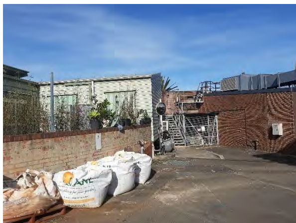
Figure 30 – Rear of existing reptile house with services evident. Aspect: south.
