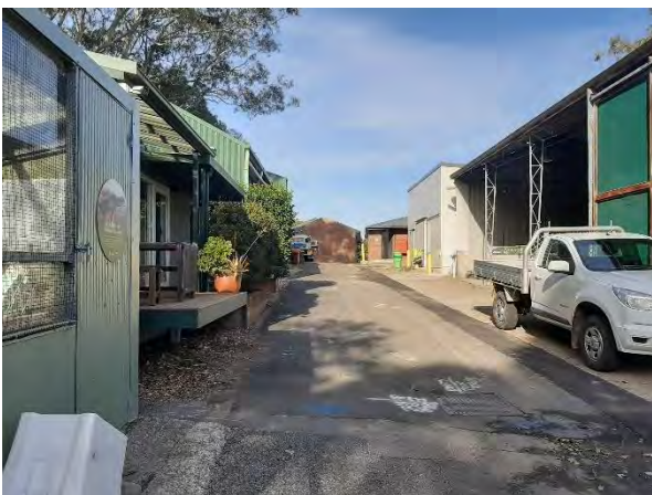
Figure 26 –General view, back of house area, with services evident. Aspect: north.
