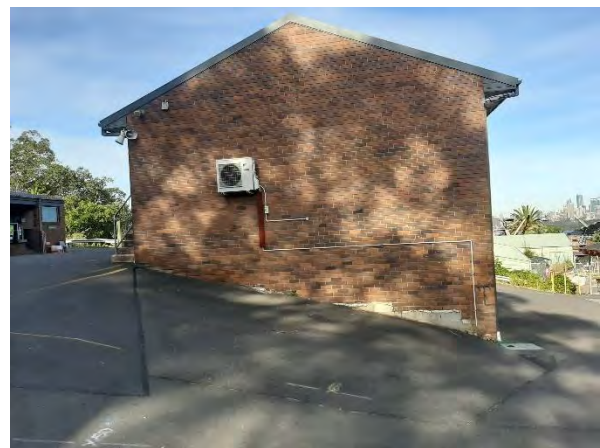
Figure 27 – Building cut into modified landscape. Aspect: south.
