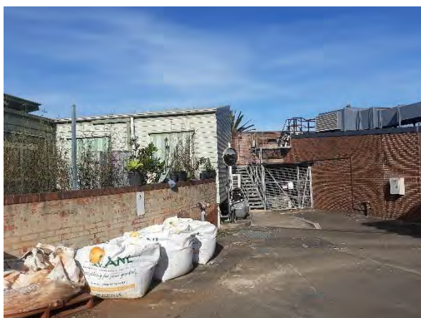
Figure 7 – Rear of existing reptile house with services evident. Aspect: south.
