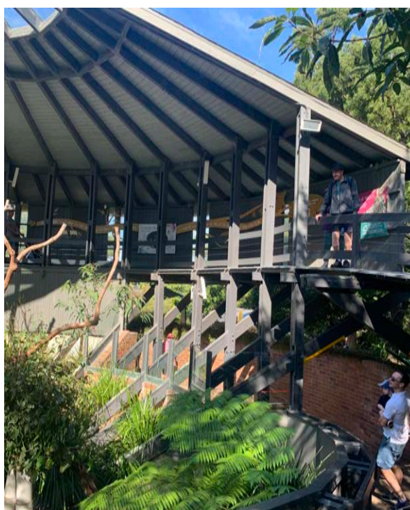
Figures 57 LEFT and 58 RIGHT Views from within the Koala House showing part of the double helical walkway system that enables views of the koalas from different perspectives. The sophisticated, yet compact cantilevered timber structure supporting and unifying the deck and roof is plainly visible, its minimal, earthy materials and vertical rhythms engaging with the surrounding trees. Owing to budgetary constraints, parts of the structure were even built by Taronga Zoo employees. (Geoffrey Britton, 2021)
