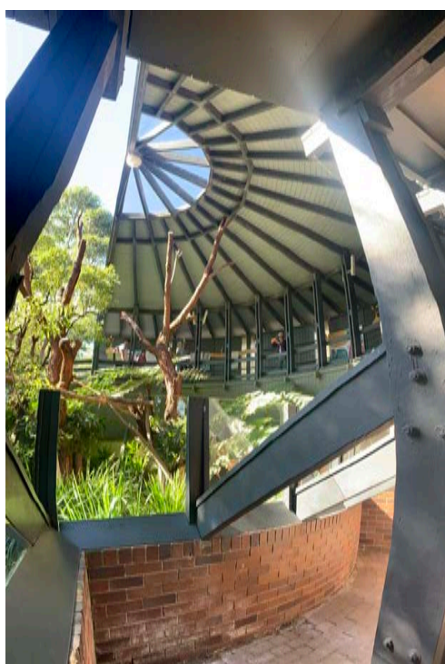
Figures 57 LEFT and 58 RIGHT Views from within the Koala House showing part of the double helical walkway system that enables views of the koalas from different perspectives. The sophisticated, yet compact cantilevered timber structure supporting and unifying the deck and roof is plainly visible, its minimal, earthy materials and vertical rhythms engaging with the surrounding trees. Owing to budgetary constraints, parts of the structure were even built by Taronga Zoo employees. (Geoffrey Britton, 2021)
