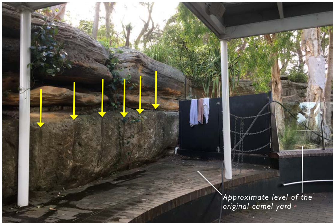
Figure 63 View of the northeastern teaching space looking into the back of the Freshwater Crocodile enclosure showing the retained approximate level of the former camel yard with the 1910s drill marks in the rock outcropping (arrows) to blast away the former stone projections. (Photograph: Jean Rice, 2022)
