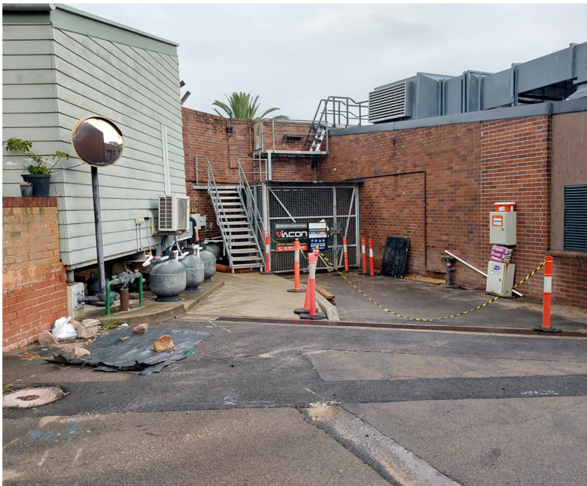
Figure 3.4 Existing Stormwater Drainage Infrastructure (Grate West of site) which is to be upgraded
