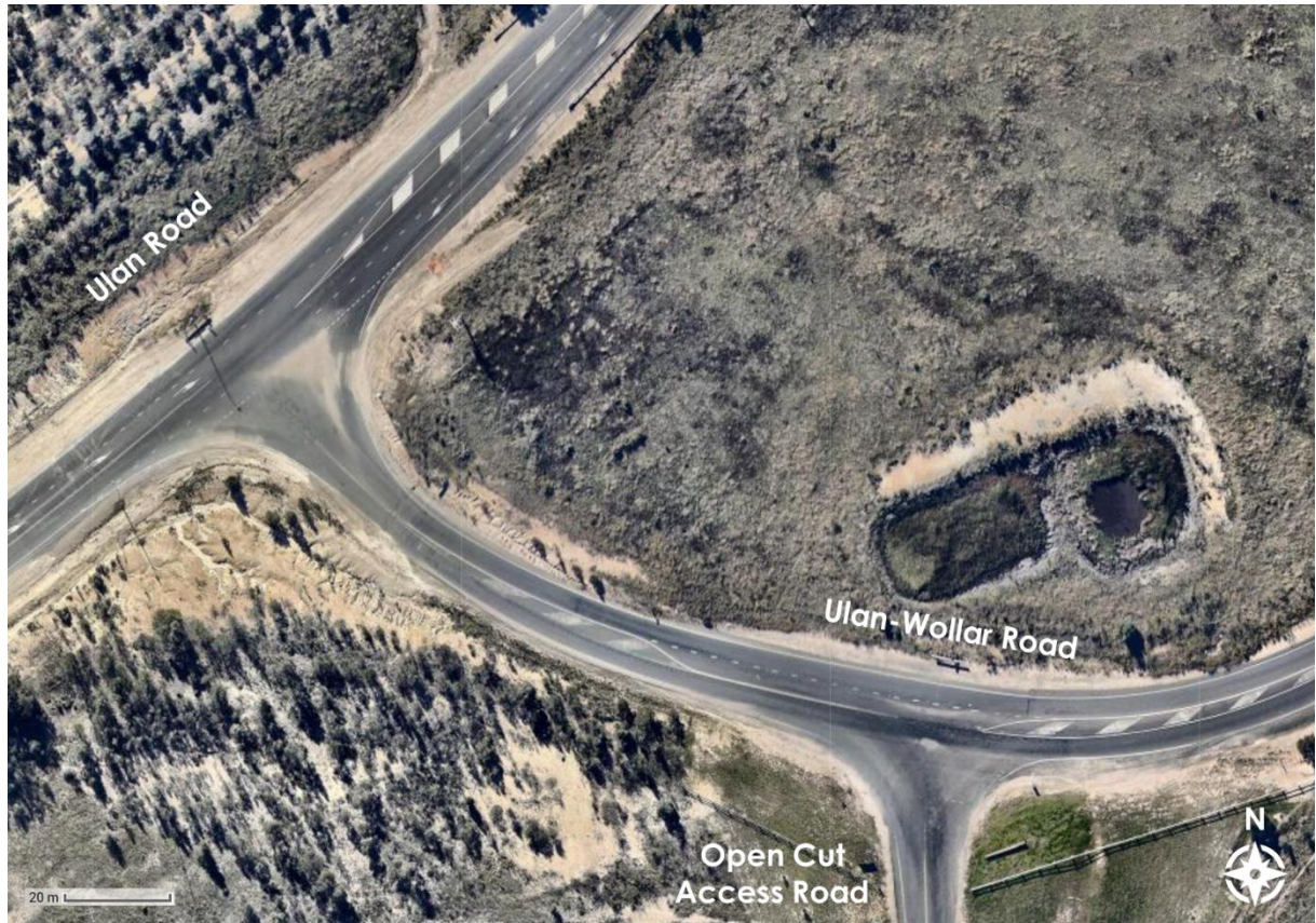
Figure 3.2: Ulan-Wollar Road at Ulan Road and Open Cut Access Road Intersections
