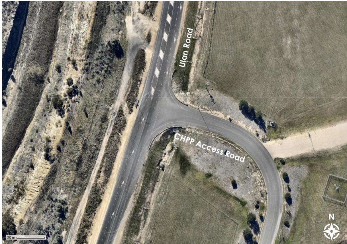
Figure 3.1: Ulan Road and CHPP Access Road Intersection
