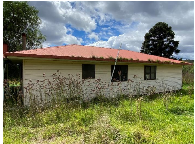
Plate 10 Abandoned house within the south- eastern portion of the Subject area.
