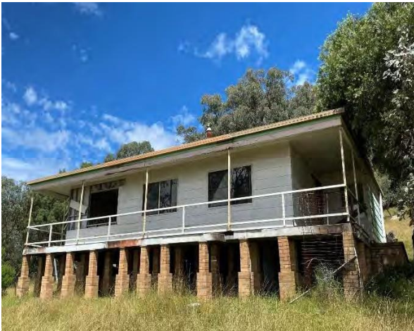
Plate 9 Abandon residence showing brick coursework stumps and verandah, in the south-eastern section of the Subject area.
