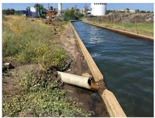
Photo 2-9 Buried ACM pipe observed on channel bank (March 2021)
