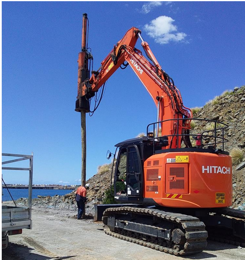
Figure 3 Impact Piling rig with Pile
