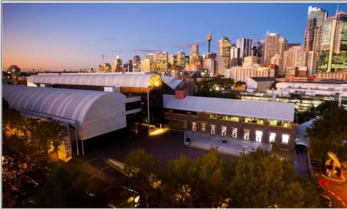
Figure 3 | Existing buildings on the site including the Wran Building (left), Switch House (right) and heritage core behind (Source: EIS)
