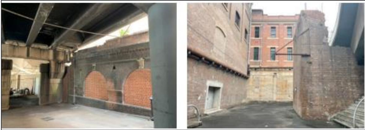
Figure 16 | Remains of the former Pump House (Source: Applicant's HIS)
