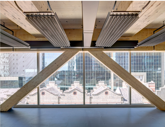
Daramu House CLT Structure, Tzannes Image credit: Brett Boardman
