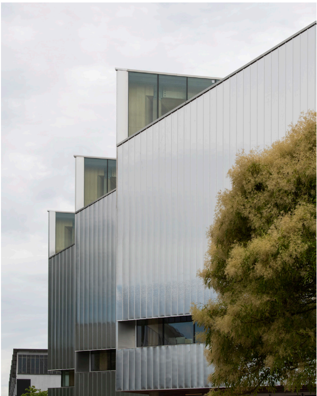
UTAS Inveresk Library recycled aluminium facade, John Wardle Architects Image Credit: Anjie Blair
