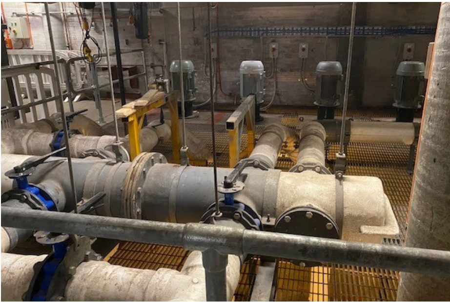
Figure 16.9 Sea Water pump pit suction motors (Source: Powerhouse)
