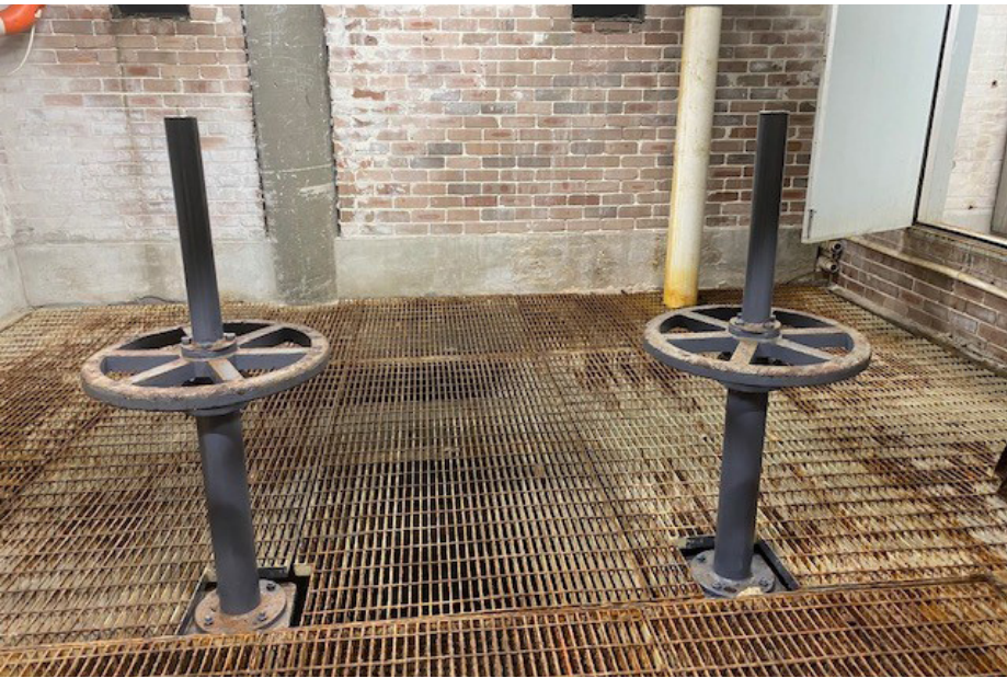
Figure 16.8 Sea Water pit and penstock valve (Source: Powerhouse)
