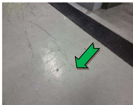
30. Interior, roof level, lift motor room, floor – non lead-containing grey upper paint system
