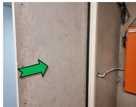
12. Interior, level 6, air handling room, door lining – non asbestos-containing fibre cement sheet
