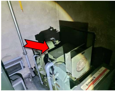
19. Interior, lower B2 level, lift motor room 3, lift motor – assumed asbestos-containing friction pads
