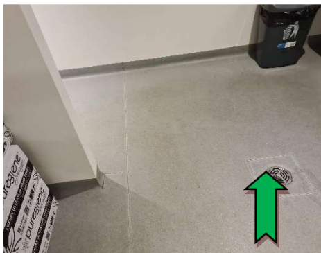
17. Interior, level 1, western elevation, Sydney Symphony Orchestra tenancy, bathrooms, floor – assumed non asbestos-containing sheet vinyl
