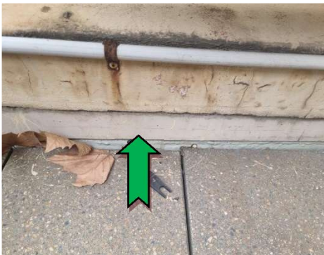
5. Exterior, level 4, balcony, base of perimeter walls – non asbestos-containing bituminous material
