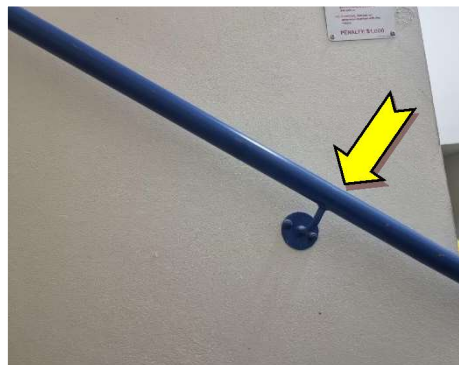
28. Interior, level 2, northern elevation fire stairs, handrail – lead-containing blue upper paint system
