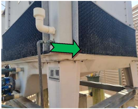
1. Exterior, roof, aqua cooling towers, base of tower, below vents – non asbestos-containing mastic sealant
