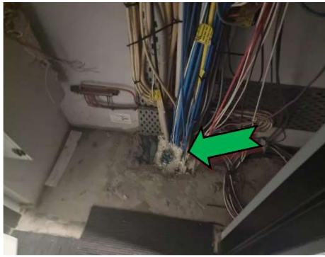
13. Interior, level 5, southern riser cupboard, under pipe penetrations – non asbestos-containing mastic material
