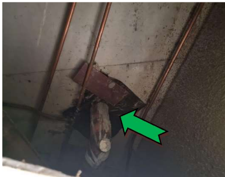
15. Interior, level 3, tea room, ceiling space, pipe penetration wrap – non asbestos-containing bituminous material
