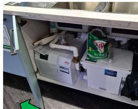
18. Interior, south west elevation, Sydney Symphony Orchestra tenancy, kitchenette – non asbestos-containing grey floor coverings
