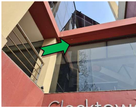
9. Exterior, level 1, north eastern elevation, below Clocktower, eave – non asbestos-containing fibre cement sheet
