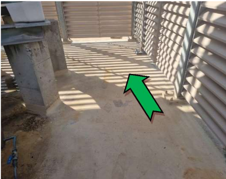
3. Exterior, roof, throughout, flooring – non asbestos-containing waterproofing
