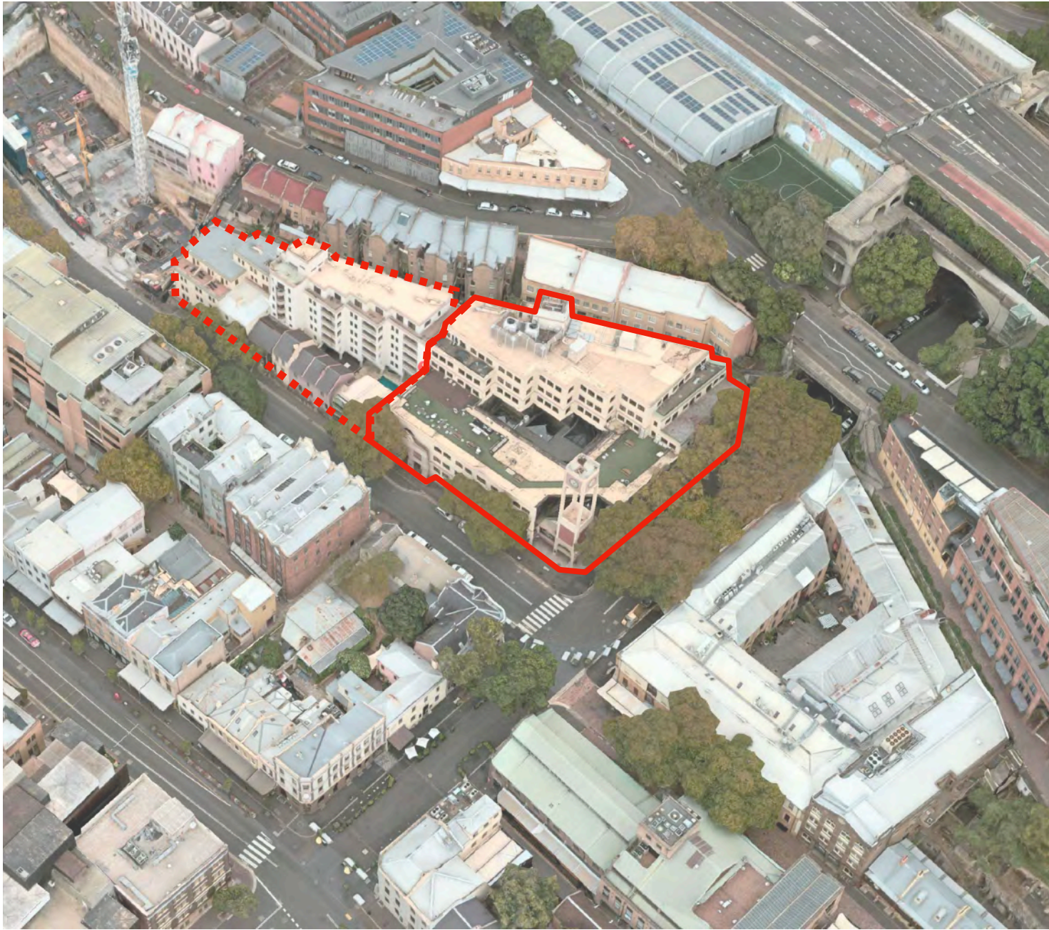
Northeast aerial perspective identifying 35-55 Harrington and 75 Harrington Street in context.
