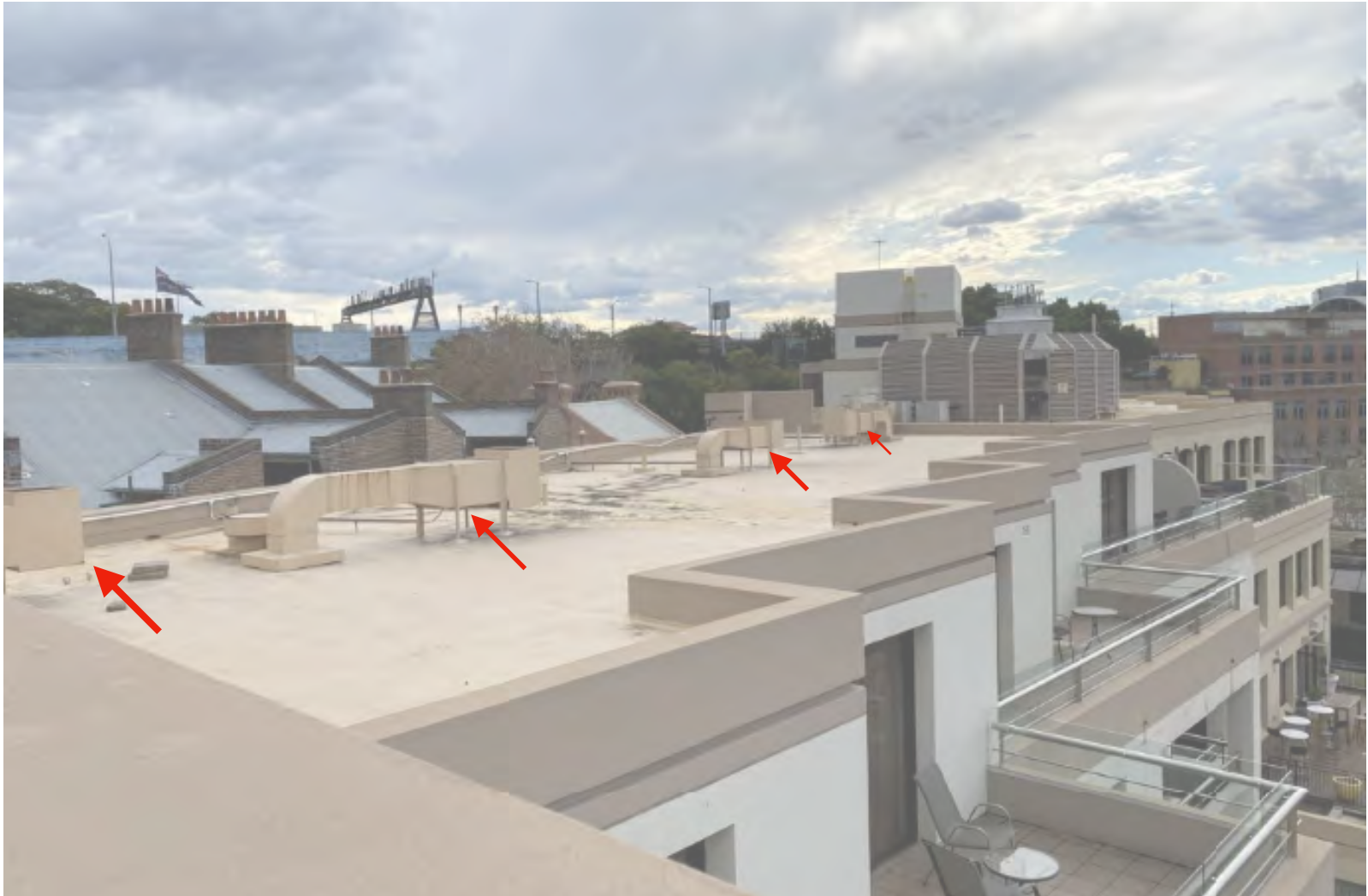
Photograph of additional rooftop plant equipment and parapet above SCRA control envelope
