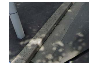
Harrington and Argyle Street Sandstone kerb and gutter
