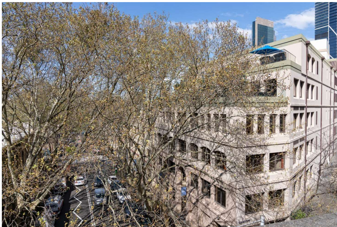
Figure 39 Argyle Bridge - existing view
