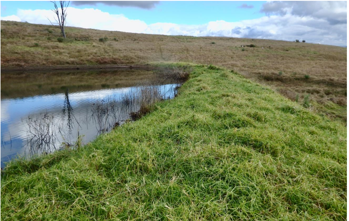
Photo 13 The main farm dam wall on Lot 35 – an artificial structure dominated by pasture grasses and weeds and lacking significant native habitat or resources
