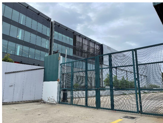
Picture 6 Data centre building to east
