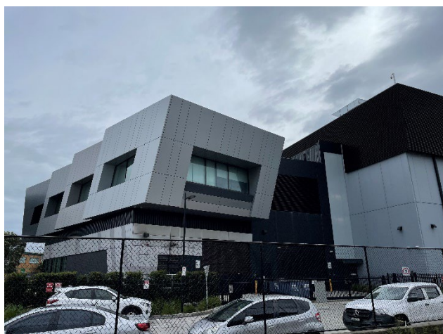
Picture 5 Data centre building to north
