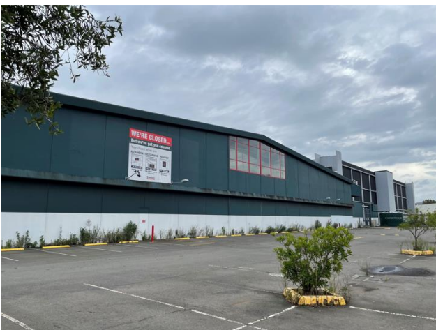
Figure 14 – Gardeners Road elevation of existing building on subject site.
