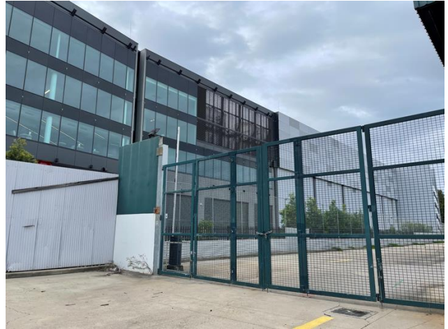
Figure 11 – Adjacent development to the east of the subject site.
