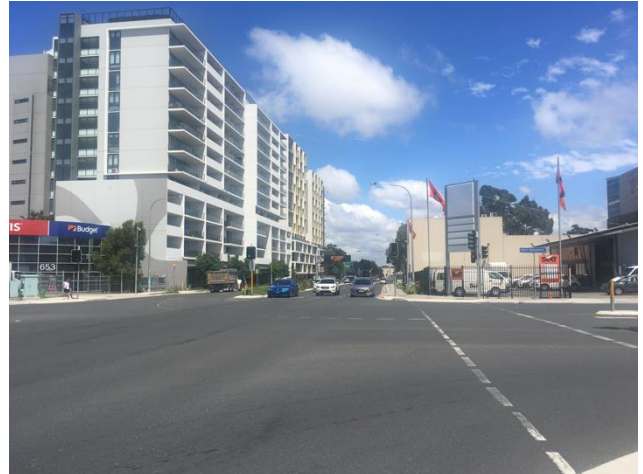
Figure 5 – Looking west along Gardeners Road.
