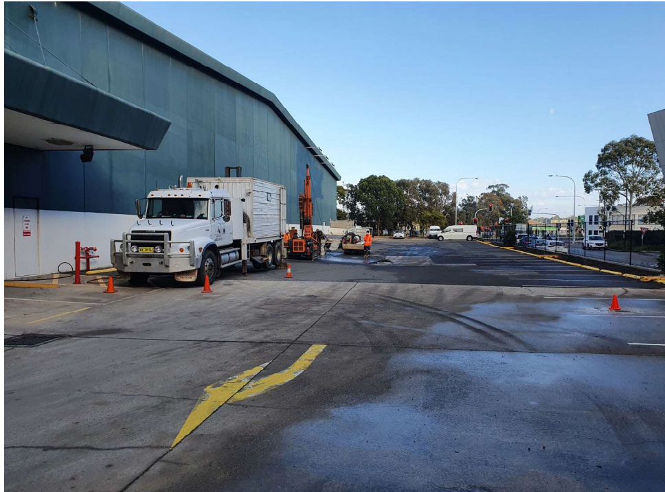
Photo 1 - Site general conditions facing west showing CPT01 & BH01 locations
