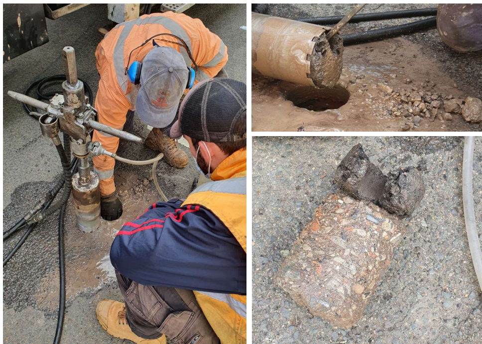
Photo 2 - Diatube coring in the location of CPT01
