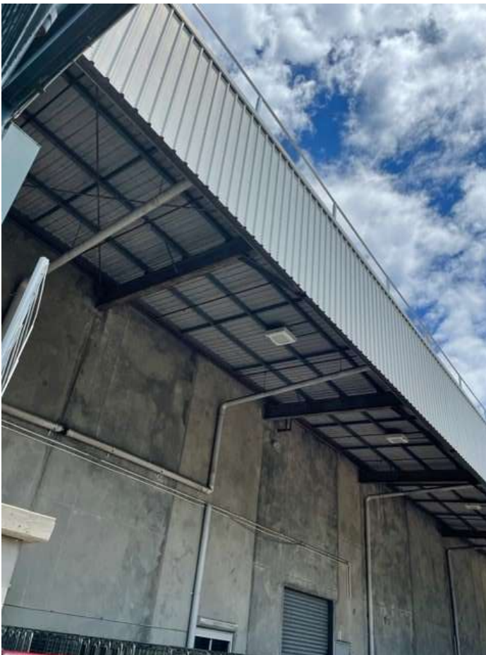
Photo 4 Building profile shows no obvious roosting habitat for microbats.
