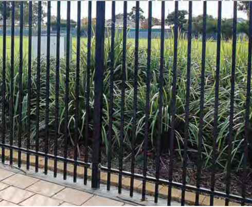
2.1m High fixed palisade fence set back 1.5m to allow planting next to footpath
