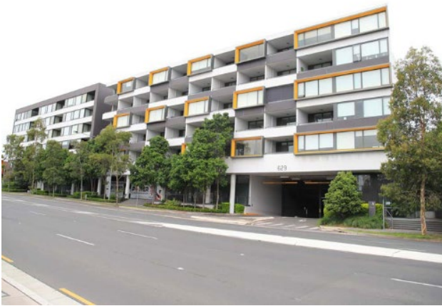
Picture 3 View of 629 Gardeners Road to the south-east of the subject site
