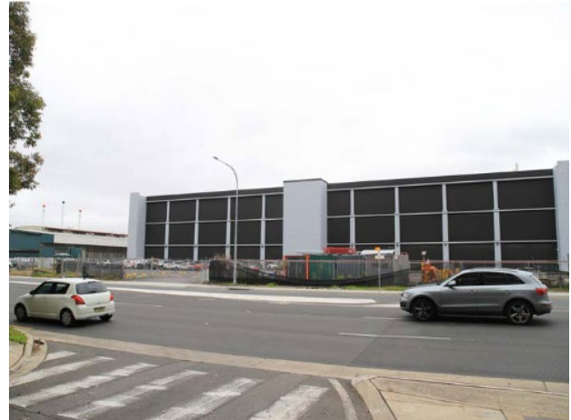
Picture 2 View north to southern elevation of the data centre at 506 Gardeners Road
