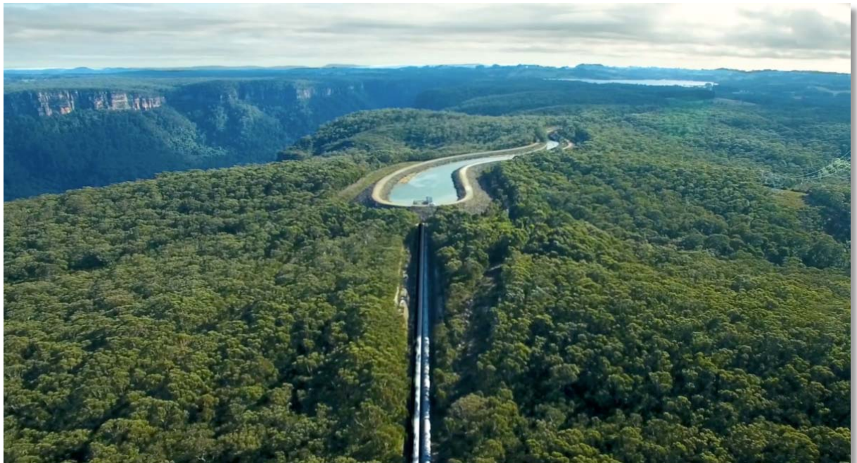
Figure 3-3: Example of a surface penstock associated with the Shoalhaven Pumped Storage Hydro Project (NSW). Note: The Central West Project will have a single penstock, not two as shown in this example (Source: ARENA, from PV Magazine , September 2019).
