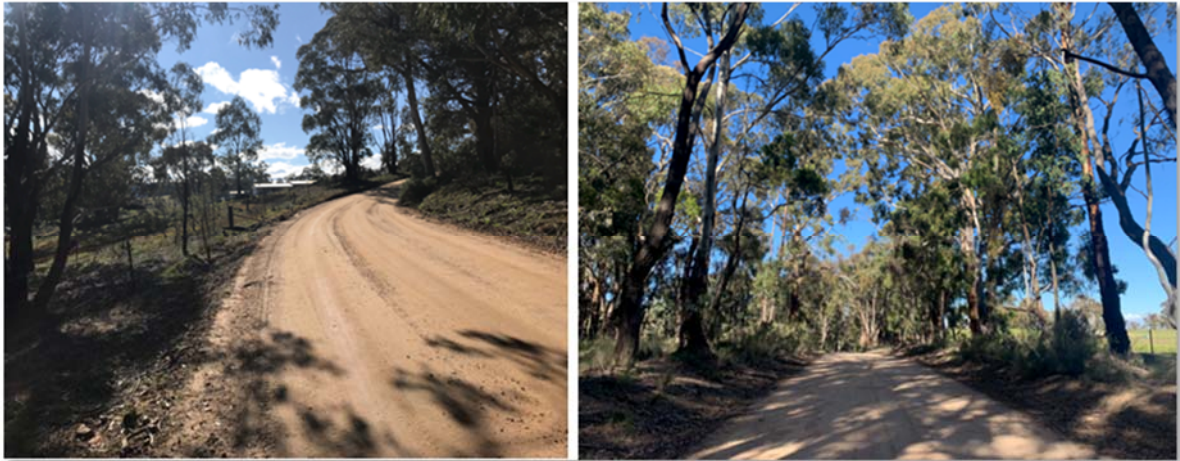
Figure 6-7: Views along Molybdonite Road.
