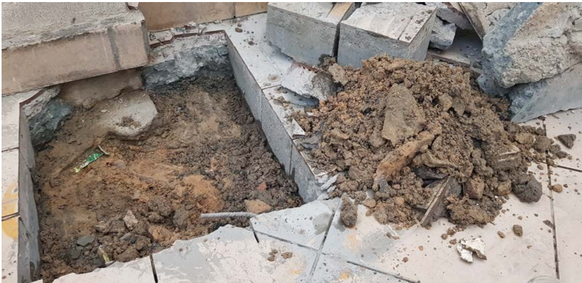
Photograph 3: General fill material across the site (5/10/2021).
