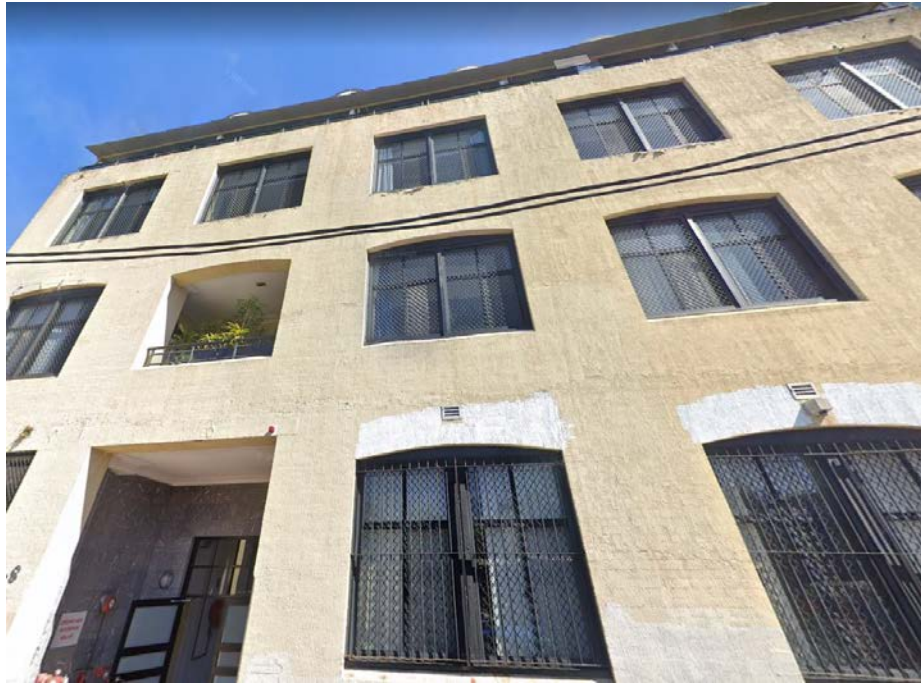
Photograph 1: Current site building, view from Woodburn Street towards west (5/10/2021).
