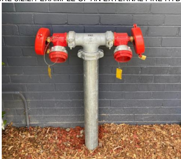
DIMENSIONS IN MILLIMETRES FIGURE 3.2.2.1 EXAMPLE OF AN EXTERNAL FIRE HYDRANT
